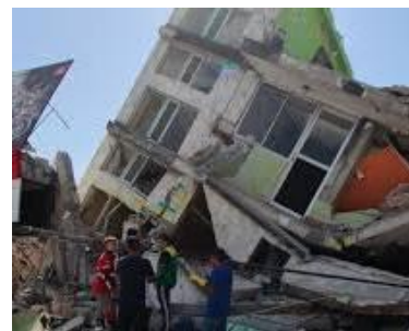
(c) Collapse of a multi-storey mixed residential building in Plaza de Bolívar 24
