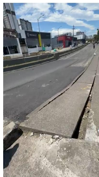
(c) Calle 17 bridge
