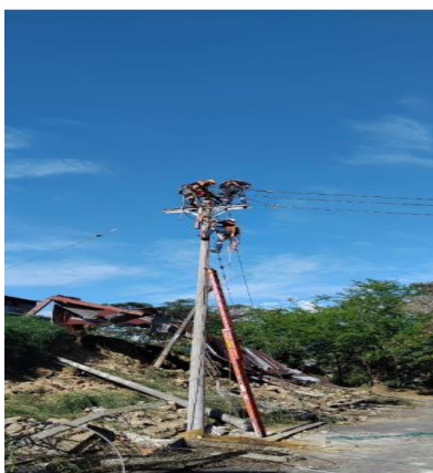
Figure 47 Pereira, Risaralda power repairs 59
