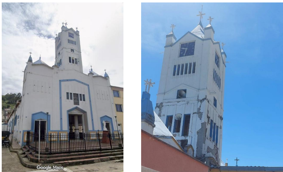
Figure 22 Iglesia La Inmaculada Concepción; before (left photo) and after (right photo) earthquake.
