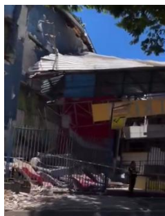
(b) Partial roof and façade collapse of a Centro Commercial Fiducentro
