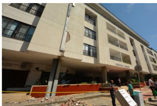
Figure 9 Amalfi RC building, Cali, Colombia, serious structural damage due to pounding movement between adjacent blocks 3 .
