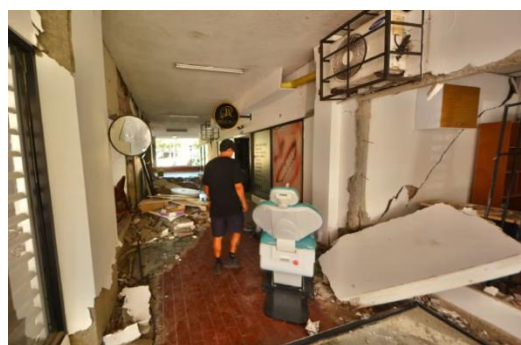
Figure 9 Amalfi RC building, Cali, Colombia, serious structural damage due to pounding movement between adjacent blocks 3 .
