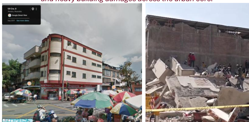
Figure 29 The collapse of Edificio Villa in Pereira; before (left photo) and after (right photo) earthquake 28
