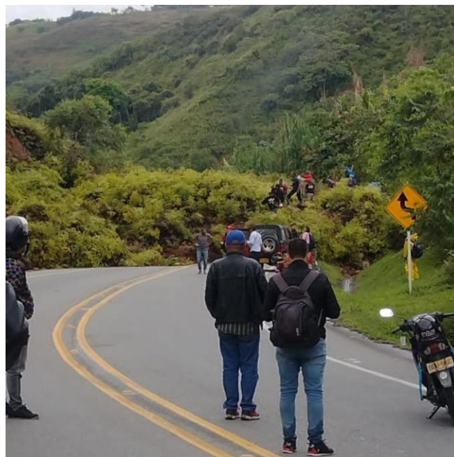
Figure 41 Landslide along the Armenia-Pereira-Manizales corridor. 53
