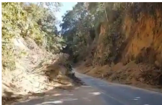
Figure 38 Landslide along the Armenia-Pereira-Manizales corridor. 43
