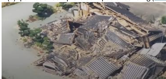
(c) complete collapse of building ( Link 70 )
