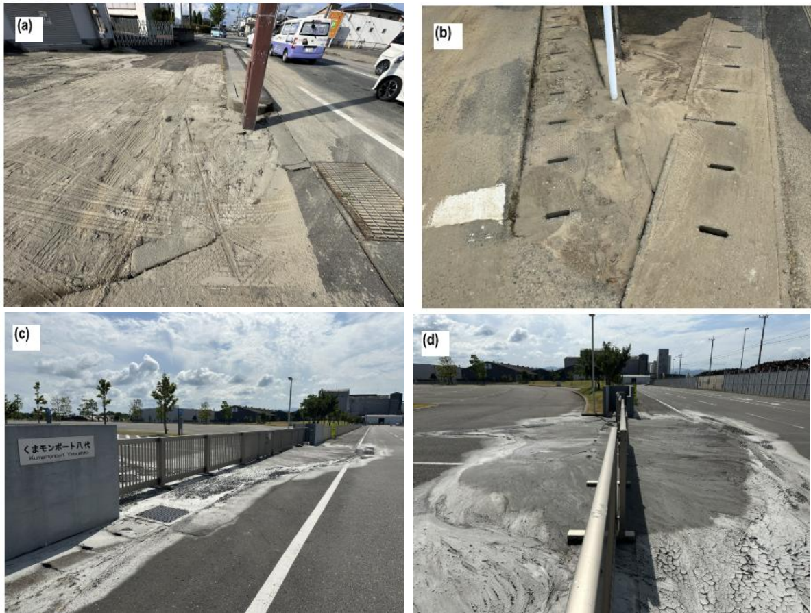
Figure 15 Sand ejecta (following liquefaction) observed at (a) Near 149-15 Tomiimachi Sugijima, Minami Ward, Kumamoto 21 (b) Yatsushiro Castle 22 (c) & (d) Yatsushiro Port 23 (refer Figure 25 for aerial imagery)
