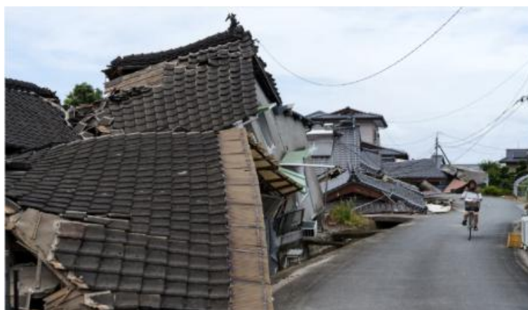
(e) complete collapse of building ( Link 72 )
