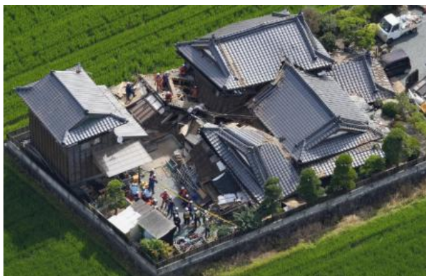
(a) partial or complete collapse of building ( Link 69 )
