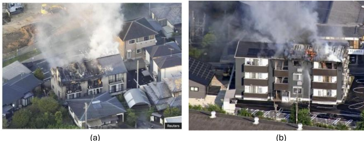
Figure 41. Fire damage to residential buildings (a - Link 74 and b - Link 75 )
