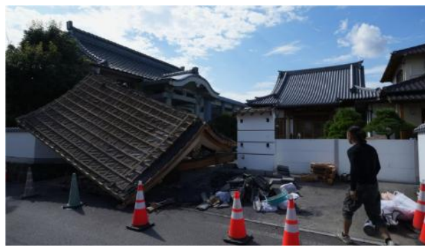
(b) After earthquake ( Link 64 )
