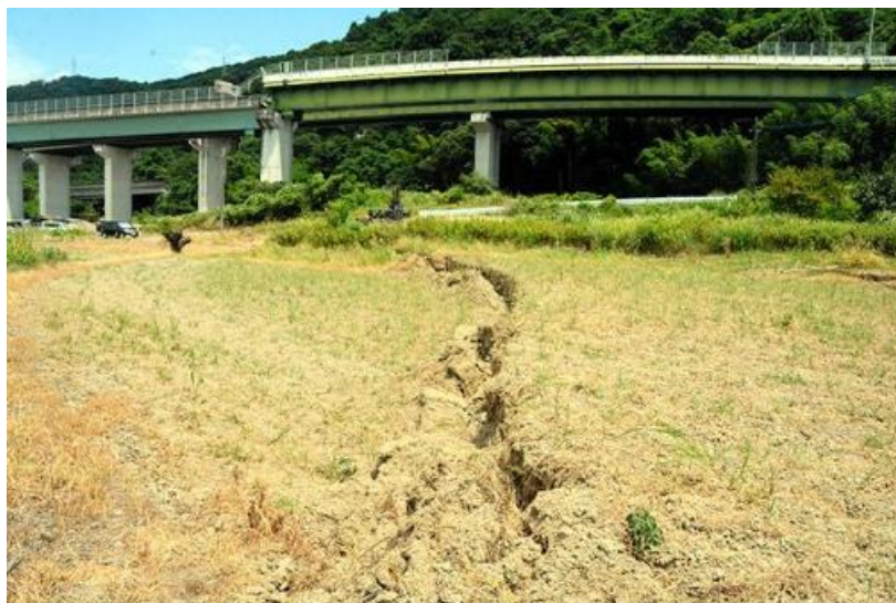
Figure 46. Ground on right side of fissure near the damaged expressway was raised by about 1 meter in Yatsushiro, Kumamoto Prefecture ( Link 92 )
