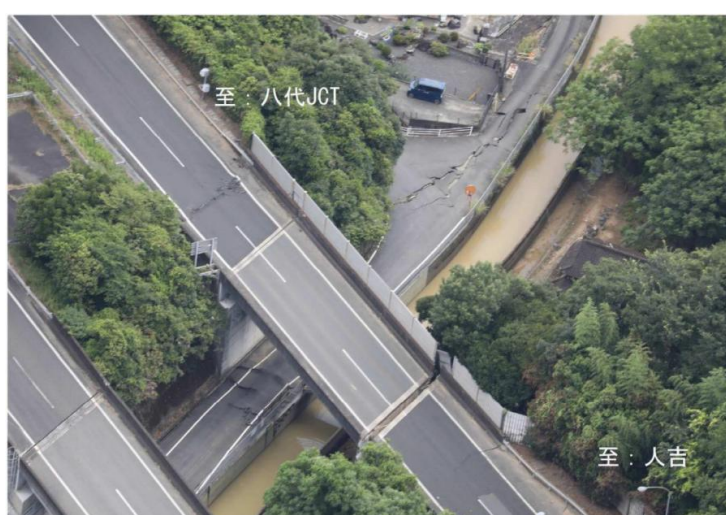
Figure 49. Damaged Katanogawa bridge ( Link 96 )
