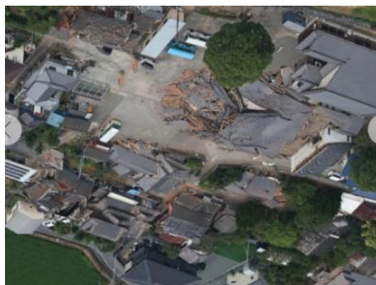
(b) After earthquake ( Link 65 )
