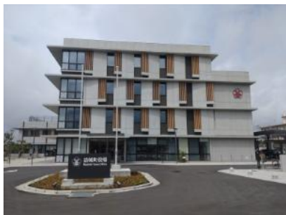
(a) Overall appearance of replaced Mashiki Town Hall [link 84 ]
