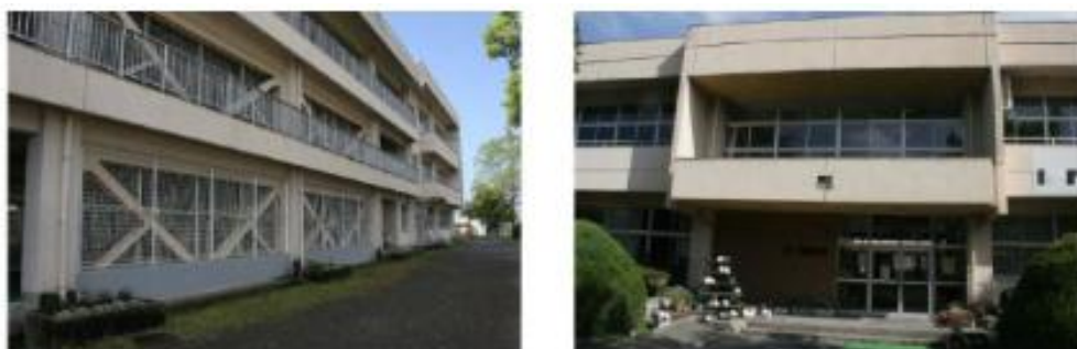
Figure 45. Kiyama Junior High School classroom blocks; external steel braces are visible on the north elevation [ link 80 ]
