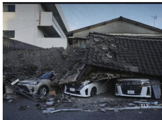
(b) roof collapse ( Link 69 )
