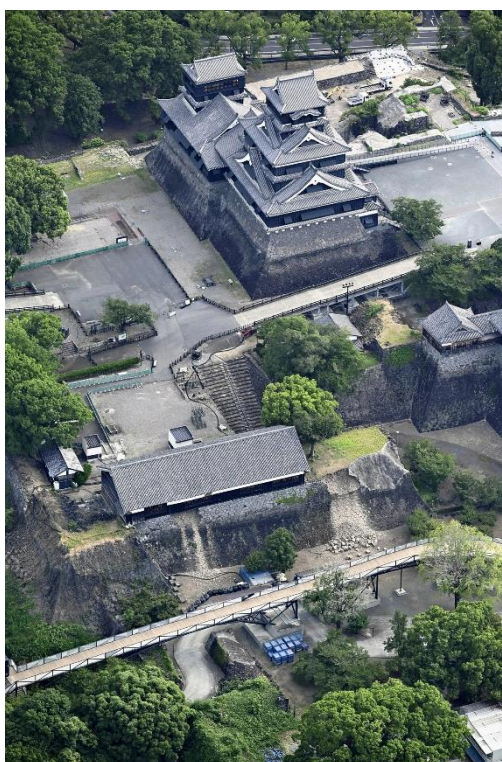
Figure 22. Kumamoto Castle with collapsed stone walls (Source: Yomiuri Shimbun 34 )
