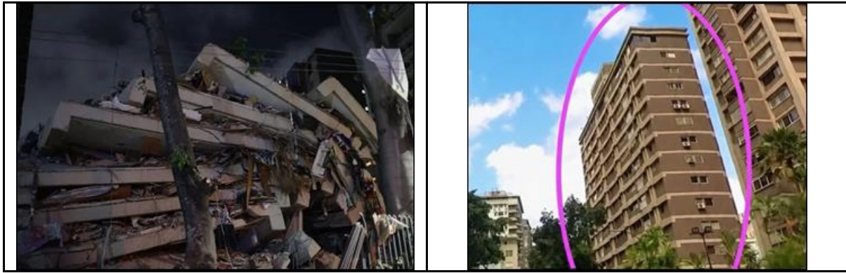
Figure 27. Edificio Petunias – a collapsed 14-storey residential RC building (left) and its original state (right).
