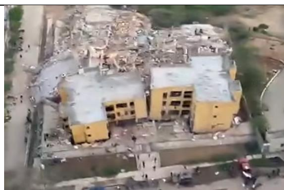
Figure 49 (right). Foundation failure evident on remaining 2 buildings at location in Catia la Mar (10.611 N, -67.011E).
