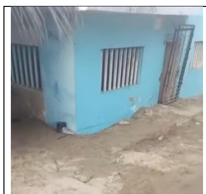
Figure 50. Liquefaction-induced settlement of a house in Boca de Aroa. (Exact position not located).
