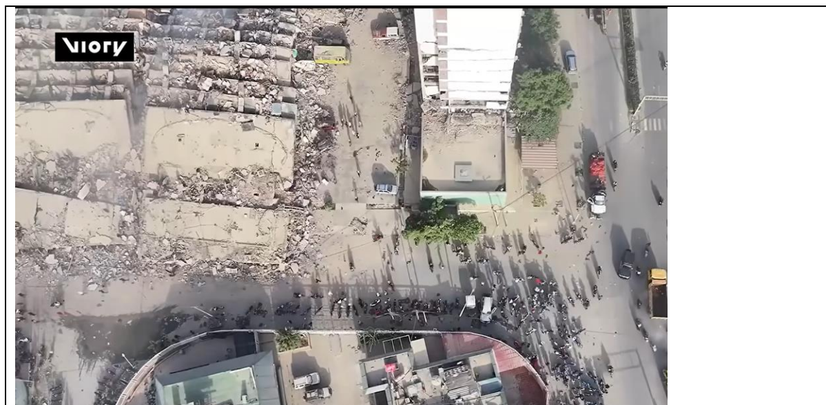
Figure 46. Overhead view in area of high damage in Carraballeda. Light coloured material on ground inferred to be from the collapse of the building rather than evidence of ejecta. (10.615N,-66.841E).
