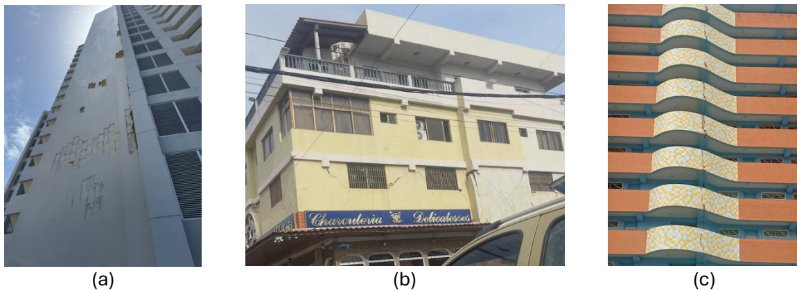
Figure 41. Architectural component damage in Tucacas: (a) detachment of facade cladding; (b) cracking of infill wall; (c) damage to elements associated with seismic separation joints.
