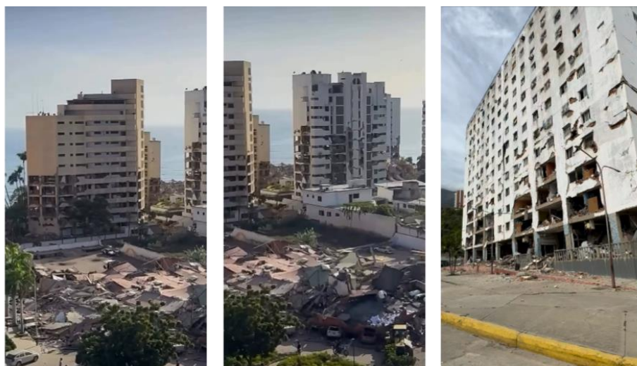
Figure 20. Typical infill damage in non-collapsed buildings (Social Media).
