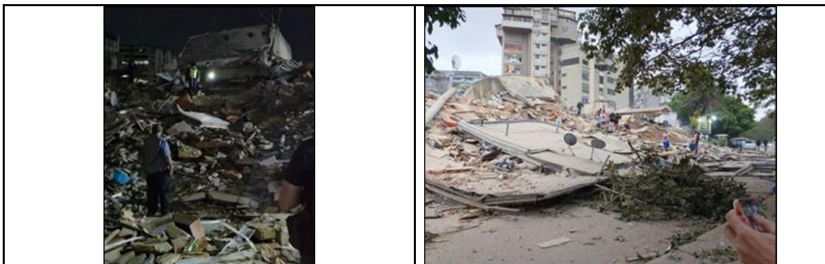
Figure 30. Edificio Rita – a collapsed 7-storey residential RC building.
