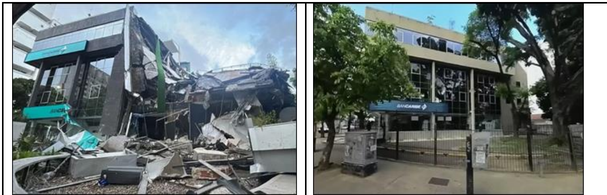
Figure 29. Edificio Bancaribe – a collapsed commercial building understood to be partially steel-framed.
