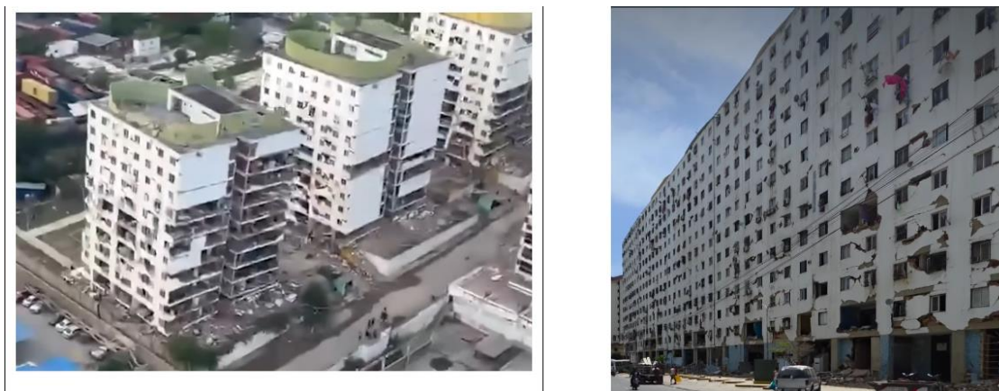
Figure 22. Government housing in Catia La Mar with collapsed ground floor (left, Social Media ) and in Caraballeda (right, Social Media ).
