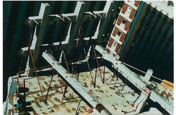
13-storey Precast Concrete Perimeter Frame office building on the Terrace, Wellington
