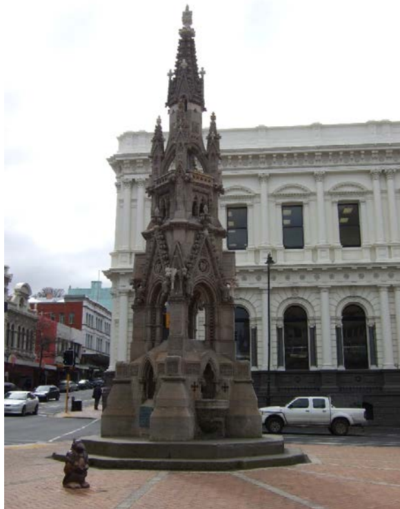
Figure 11. Restored and Strengthened Monument.
