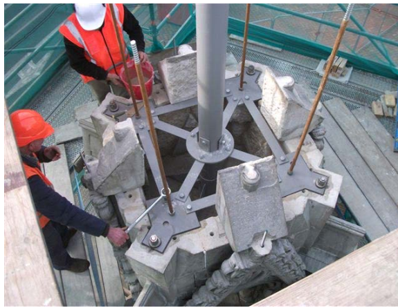
Figure 9. Re-Construction plates and rods.
