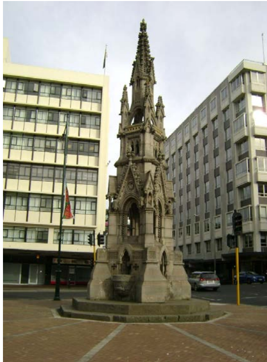
Figure 3. Cargill's Monument before restoration.
