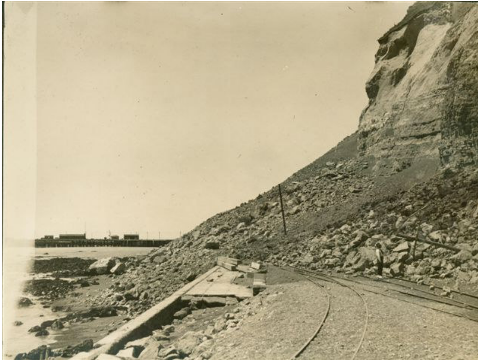
Figure 7. Damage to Napier's Breakwater Harbour and Bluff Hill obliterated parts of the road and railway line.
