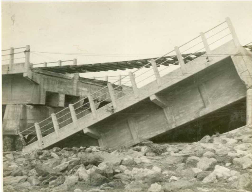
Figure 6. Damage to the Westshore Bridge, Embankment Road.
