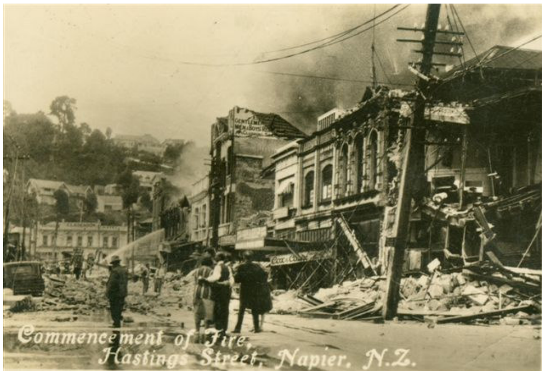
Figure 1. A critical moment: Minutes after the earthquake fire started in Hastings Street, Napier.
