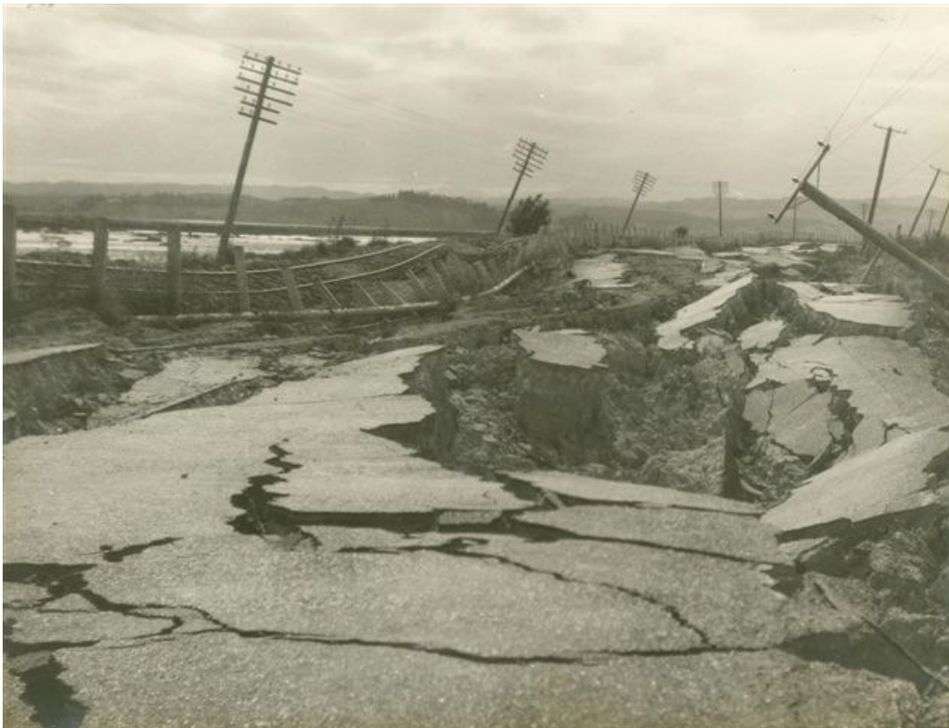
Figure 5. Damage to the rail, road, power and communications services was significant. An example of the extent of the damage can be seen in this photograph of Embankment Road in Napier.
