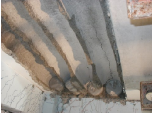
(b) Close up looking at the seat damage
