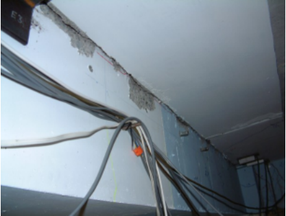
(b) Entire seat has been lost at the completion of the Phase I (-2.0% drift)
