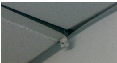
Damage caused by failure of the main beam/cross-tee to wall angle rivet
