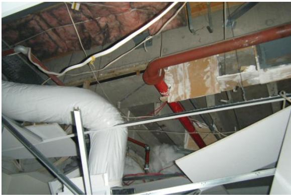
Ceiling damage in the upper floor with heavy tiles
