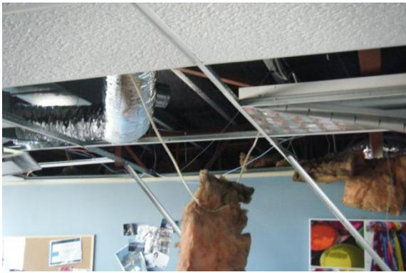
Ceiling damage caused by unbraced AC ducts
