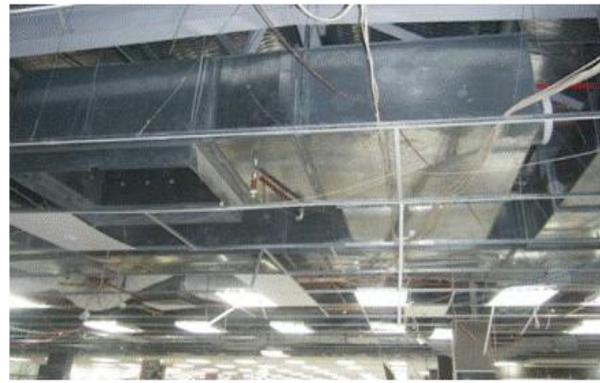
Damaged ceiling with inadequate service height
