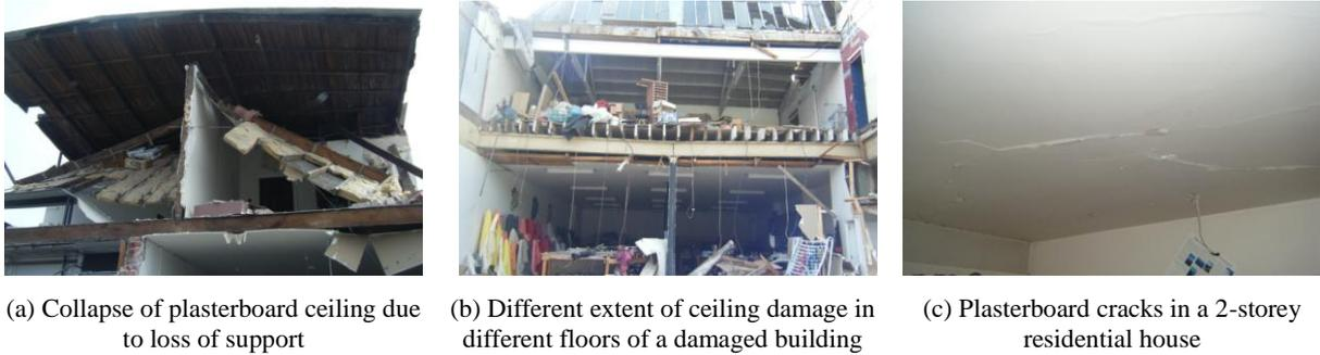
**Figure 3: Typical damage to residential plasterboard ceilings.**
