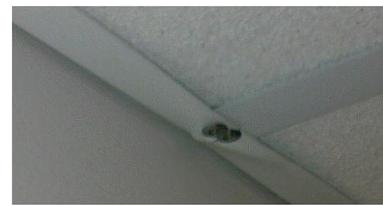
Perimeter connection with increased number and diameter of rivets
