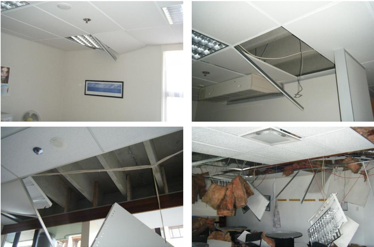
**Figure 6:** Localised ceiling damage due to failure of the grid members to wall angle connection.
