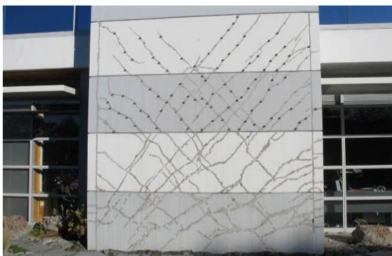
Figure 70: Crack epoxy grout injection repair for RC wall.
