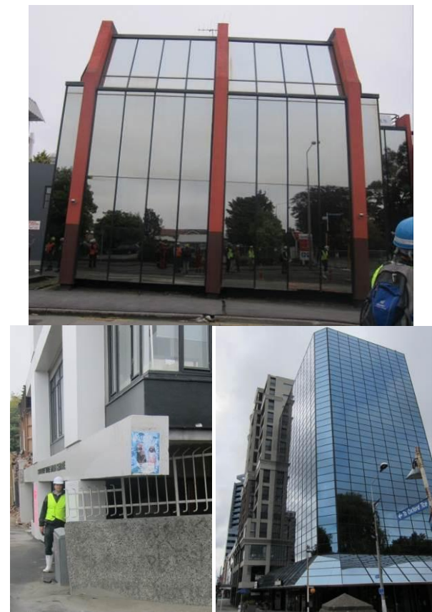
Figure 72: Liquefaction induced differential settlement resulting in significant tilting of mid- to high-rise buildings of various foundation and soil details: a) Four-storey with shallow foundation; b) Six-storey with shallow foundation; c) Two high-rise buildings with substantial differential settlement and tilting.
