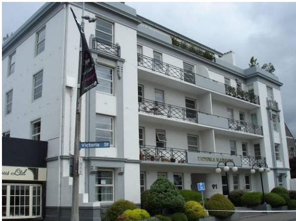
Figure 25: a) 4-storey Victoria Mansion (1935), with RC walls or possibly RC frame with infill walls, had limited structural damage; (b) 4-storey RC frame/wall National Bank / Isaac House (1926) showed limited cracking and damage from preliminary inspection.
