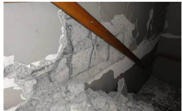
Figure 36: Failure of unconfined grouted duct splice for longitudinal bars of precast concrete walls.
