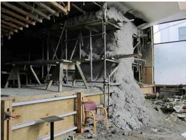
Figure 66: Concrete encasement for temporary stabilisation of an axial-shear-damaged RC wall.
