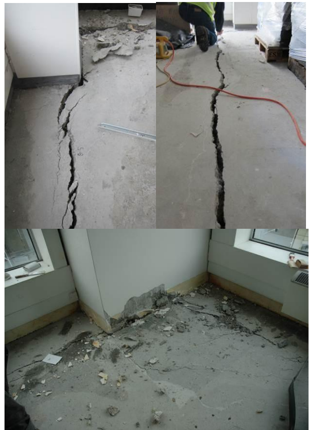
Figure 30: Extensive damage of floor diaphragm and loss of floor support for building in Figure 29 due to the beam-elongation effects of concrete frame inelastic response.
