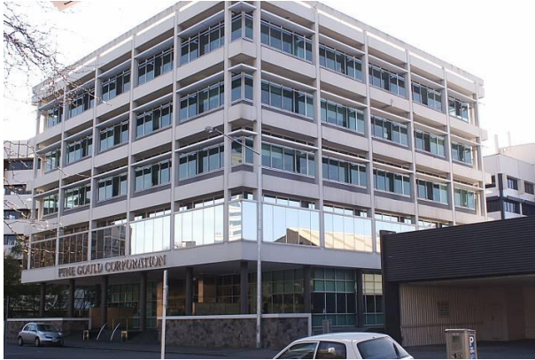
Figure 46: Pyne Gould Corp (PGC) Building photographed from the South-East elevation after the 4 September 2011 earthquake.
