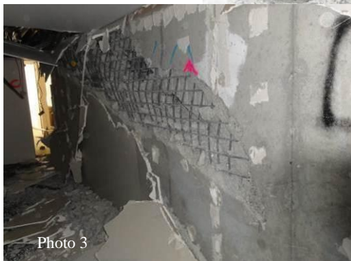
Figure 35: Boundary bar fracture and slender wall shear-axial failure in the Ground Floor of an 8-storey plus basement residential apartment building built in the 2000-2010.
