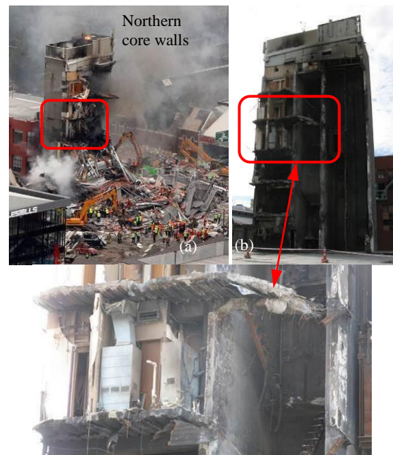
Figure 54: Northern RC core walls of the CTV Building. Photograph (a) is taken on the 23 rd February 2011 by Mark Mitchell published in New Zealand Herald. Photograph (c) illustrates the remains of the Hi-Bond floor slab deck at 3 rd and 4 th Floors.
