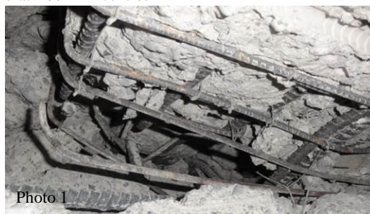
Figure 36: Failure of unconfined grouted duct splice for longitudinal bars of precast concrete walls.
