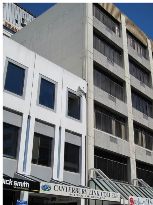
Figure 73: Pounding damage was not widely observed.
