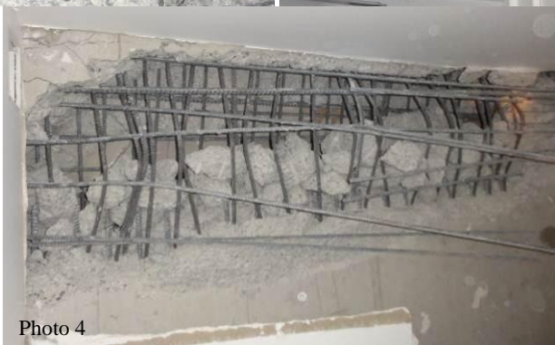
Figure 35: Boundary bar fracture and slender wall shear-axial failure in the Ground Floor of an 8-storey plus basement residential apartment building built in the 2000-2010.
