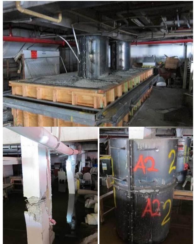
Figure 68: Emergency stabilisation repair of the basement columns with axial-shear failure.
