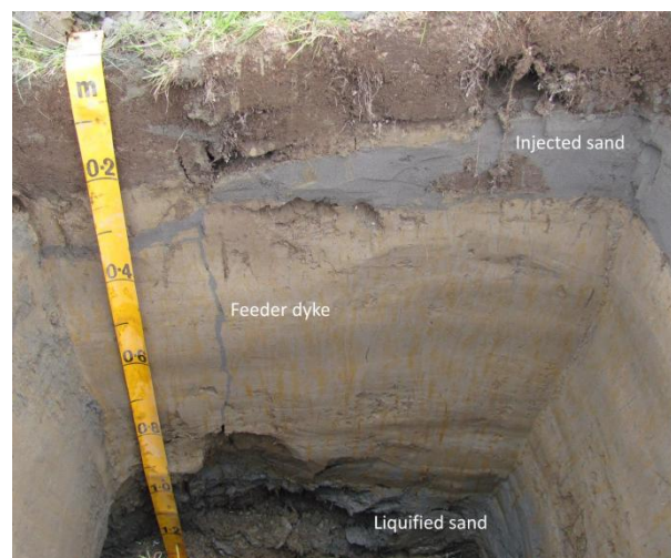
Figure 5: Soil pit exposure of a liquefaction blister. Blue-grey sand has been injected beneath the topsoil, inflating the ground surface. Note the feeder dyke from the liquefied sand beneath the water table.
