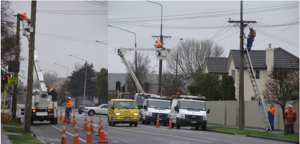
Figure 9: Linesmen at work repairing overhead lines (10 September 2010).
