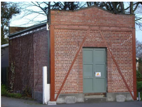
Figure 7: Zone substation with seismic strengthening.
