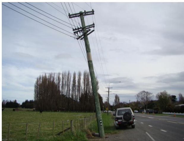
Figure 8: Lean on Pole due to liquefaction (Halswell).
