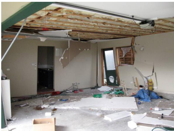
Figure 1: Lateral spreading of house in Kaiapoi.
