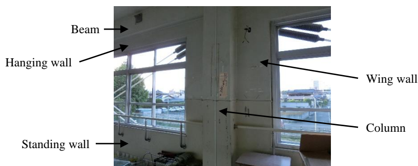
Figure 1: Photo of non-structural walls with a column and beams.
