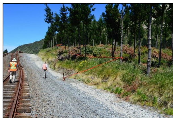
Figure 11: Surface fault rupture across a northeastern strand of the Papatea Fault near the coast deformed and distorted the SIMT line and severed the East Coast fibre optic cable at this location. Orange flagging marks the location where the fibre optic cable was cut by fault rupture and subsequently repaired (view to the southwest; photograph by Robert Zinke).
