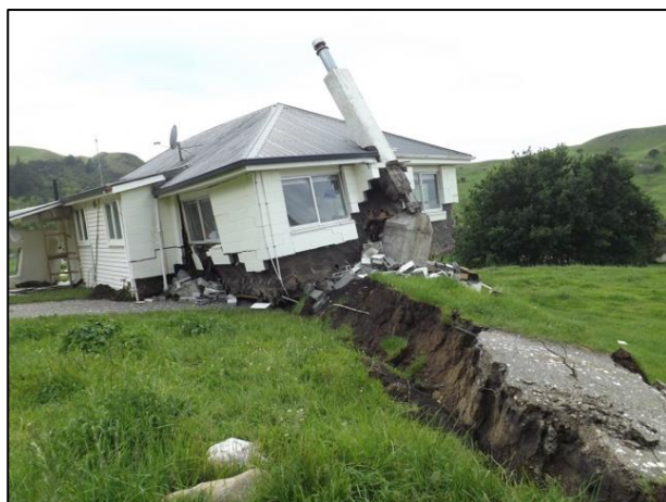
Figure 8: Direct fault surface rupture of c.8 m (dextral) through a farm worker's house across the Kekerengu Fault (Lat 41.978°S, Lon 178.998°E; view to the west; photograph by Tim Little).
