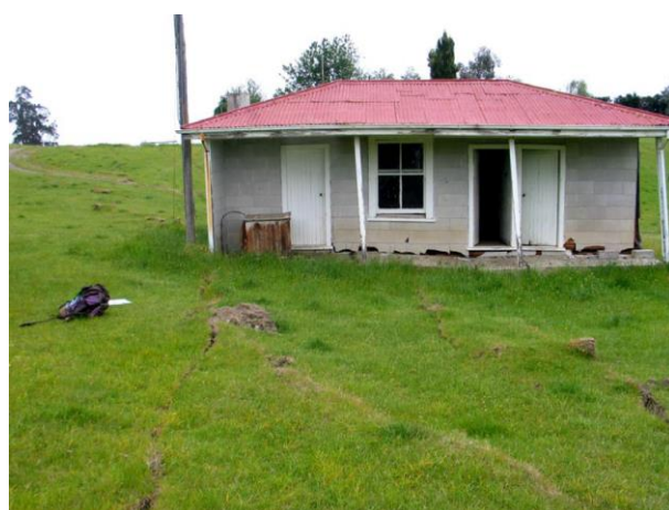
Figure 6: The Humps Fault surface rupture through a farm worker's cottage at Hossack Downs (Lat 42.629°S, Lon 173.015°E; photograph by Jarg Pettinga).
