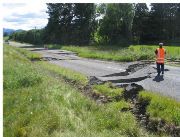
Figure 5: Oblique transtensional rupture within The Humps Fault zone displacing State Highway 70 (the Inland Kaikōura Road; Lat 42.597°S, Lon 173.091°E; view towards the north; photograph by Jarg Pettinga).
