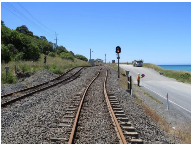
Figure 7: Dextral-reverse displacement of the SIMT and State Highway 1 across the Hundalee Fault at Oaro (Lat 42.504°S, Lon 173.510 °E). The displacement of the road was sharp, but smoothing and resurfacing was just being completed when the photo was taken. The SIMT offset was diffused through embankment ballast and the flexibility of the rails, and in this view has yet to undergo any repair or modification (photograph by Mark Stirling).
