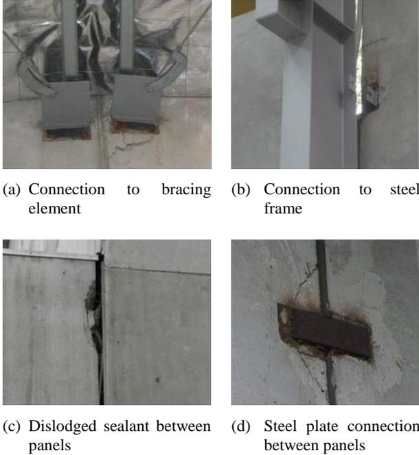
**Figure 1: Panel failures in the 2011 Christchurch earthquake [15].**
