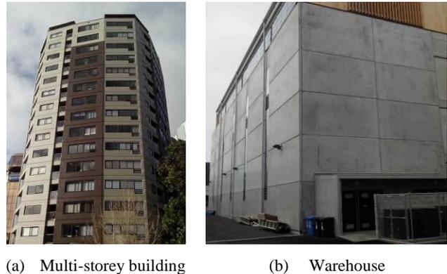
**Figure 3: Examples of precast concrete panels in New Zealand.**
