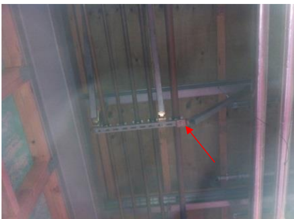
Figure 4: Cable bracing fixed to secondary steelwork and roof purlins (top); and proprietary rigid bracing in the transverse and longitudinal directions fixed to roof purlins (bottom).
