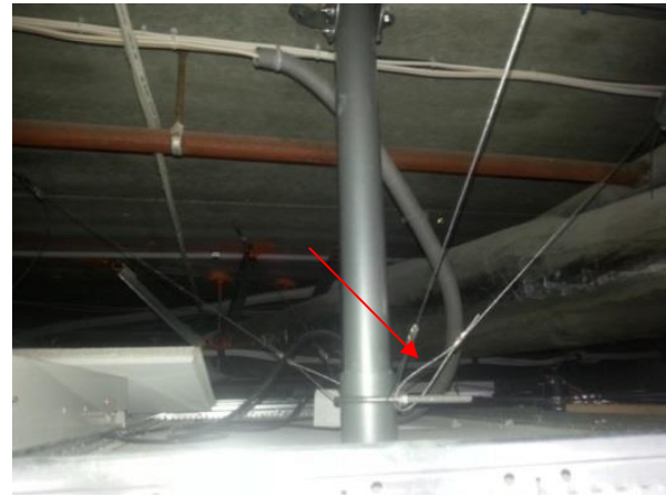
Figure 3: Wire cables added to brace A.V. equipment above ceiling level.
