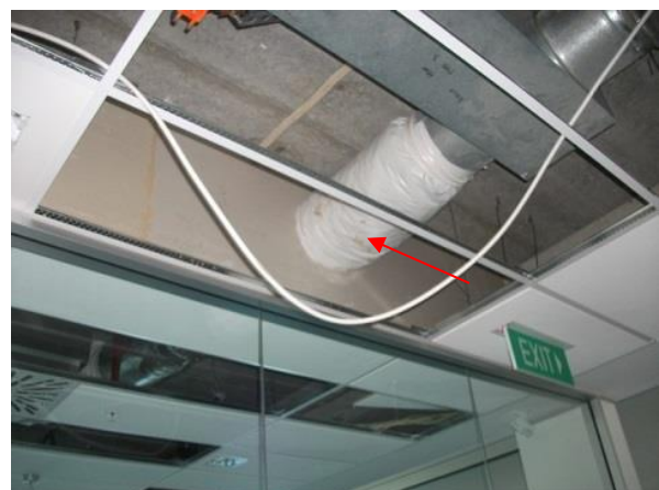
Figure 6: Rigid services passing through a wall utilising an oversized hole (top), or flexible duct (bottom).
