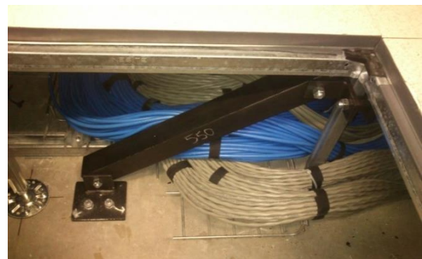
Figure 9: Sub-floor bracing added to proprietary false flooring.
