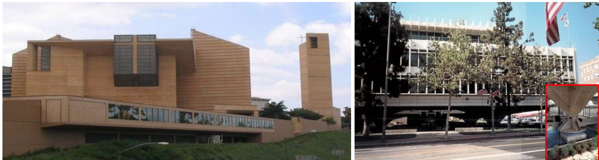
Figure 2: Example of base isolated buildings in the US: Cathedral of Our Lady of Los Angeles, Los Angeles, CA (left), Municipal Service building, Glendale, CA (right).
