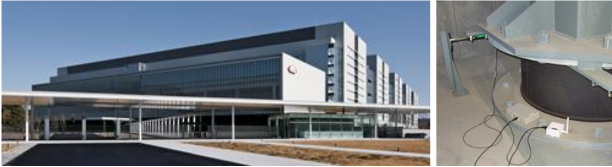
Figure 1: Example of base isolated buildings in Japan: Takeda Pharmaceutical Company Shonan Research Center, Fujisawa City, Kanagawa.
