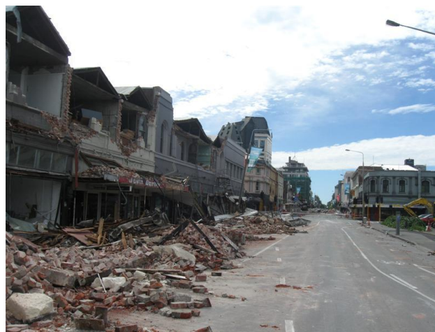
Figure 1: Out-of-plane wall collapse as a result of the 2011 Christchurch earthquake.
