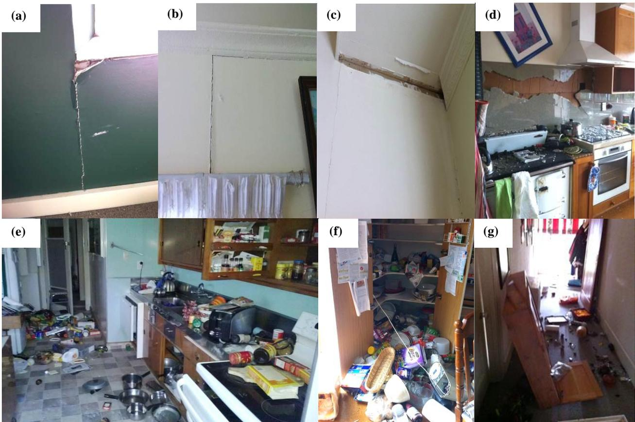
**Figure 13:** Various states of interior damage was observed: (a)-(b) wall linings; (c) detached scotia beading; (d) brittle failure of kitchen splash-backs; (e)-(g) widespread contents damage at houses located within 10 km from the fault source.
