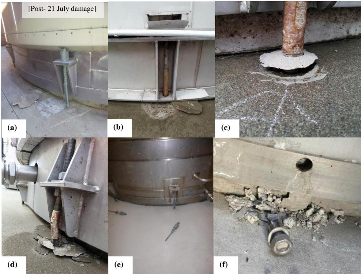
Anchorage failure by pullout, bolt tensile fracture and bolt shear failure
