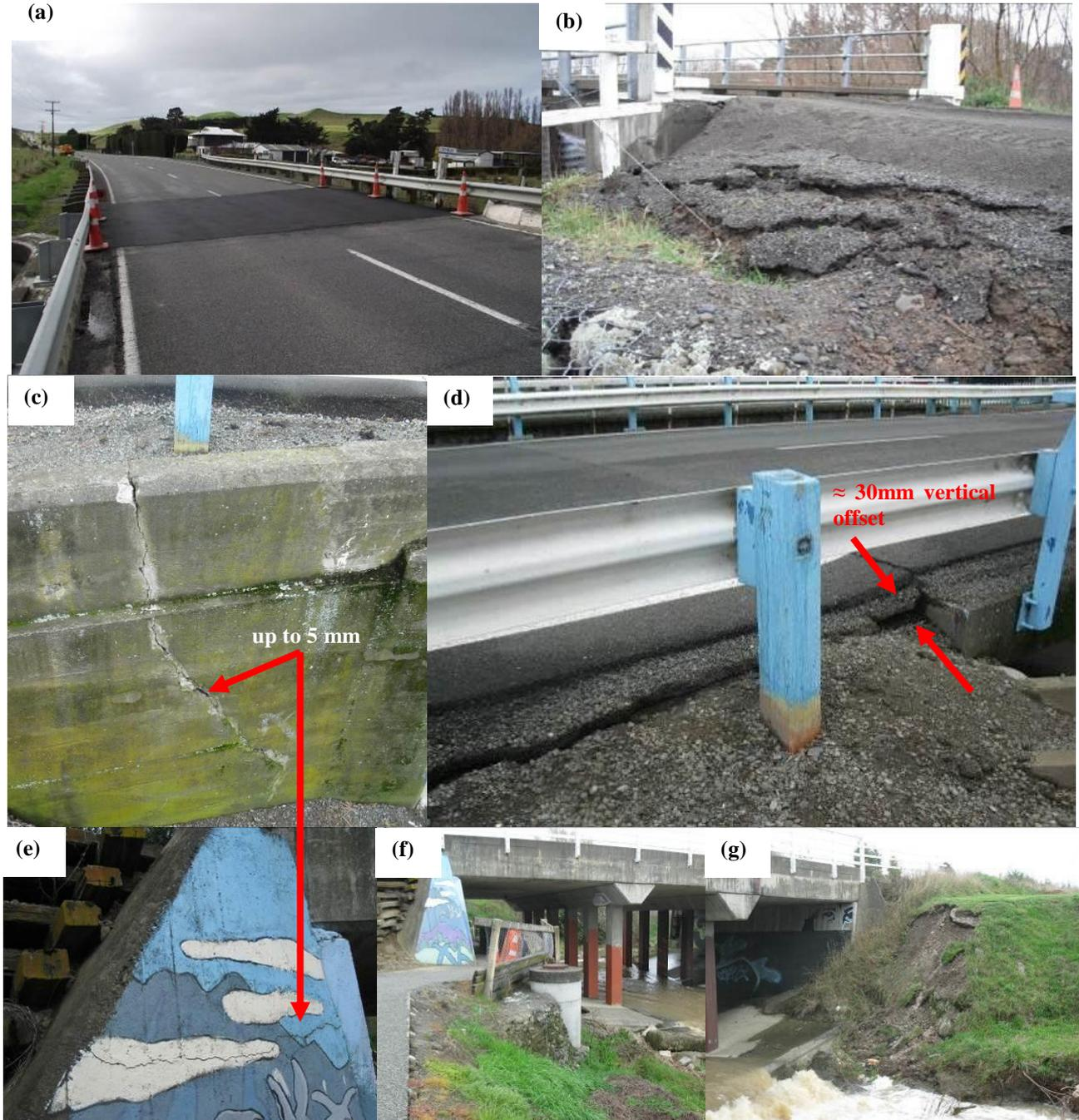
**Figure 5:** Approach settlements observed at: (a) 100 mm Needles Creek Bridge (rapid repair); (b) 400 mm Merrifields Bridge (courtesy of NZTA). Damage to road and rail bridges over the Starborough Creek on State Highway 1 included approach settlements, cracked abutment wingwalls and slope stability issues.
