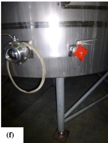
(f) Skirt and base damage to red cellar leg mounted tank
