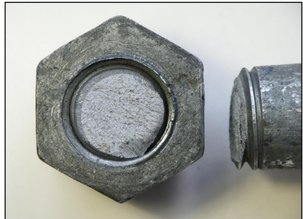
Figure 11: Failure at bar head on bridge.
