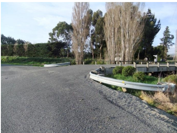
Figure 10: Remediated western approach.
