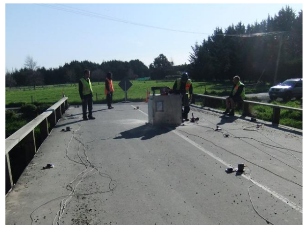
Figure 11: Shaker and accelerometers set up on bridge.
