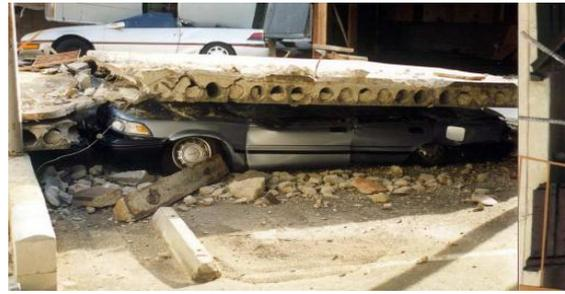
(b) Collapse of hollow-core flooring unit following 1994 Northridge earthquake (Norton et al., 1994).
