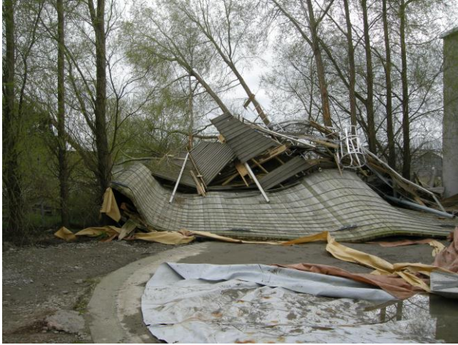
Figure 1: Total collapse of storage tanks in the Darfield earthquake (2010) (Courtesy of Timbertanks).
