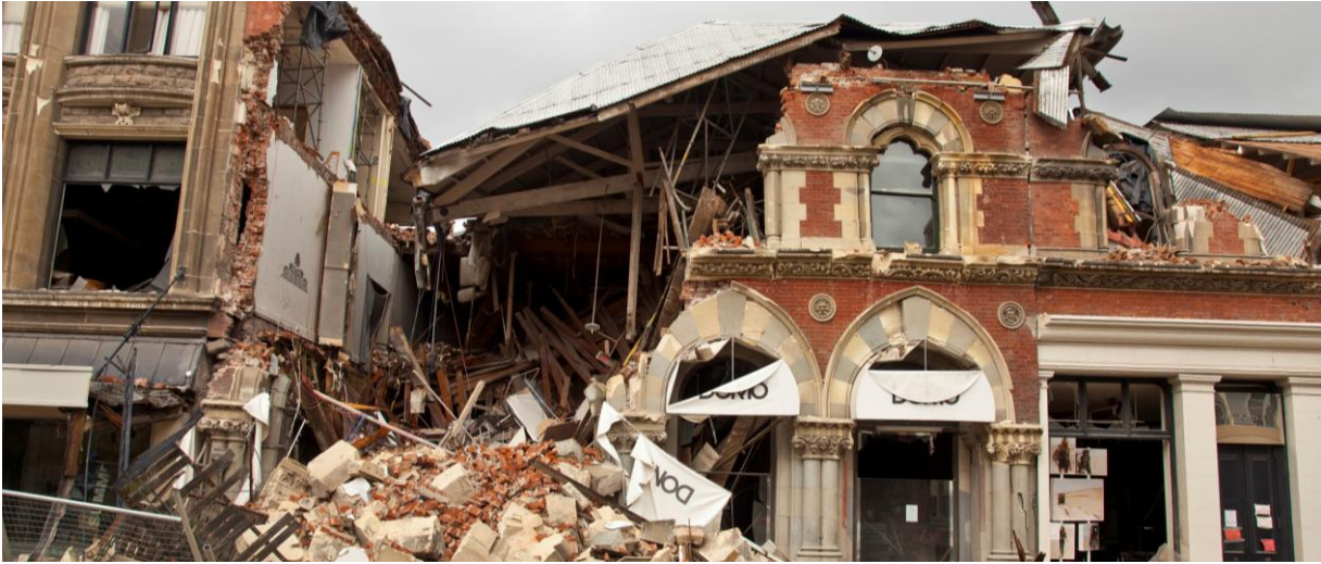
Figure 10: Building collapse involving building pounding. Primary cause of collapse is attributed to URM construction. (Photo courtesy of Colin Monteath, Hedgehog House.)
