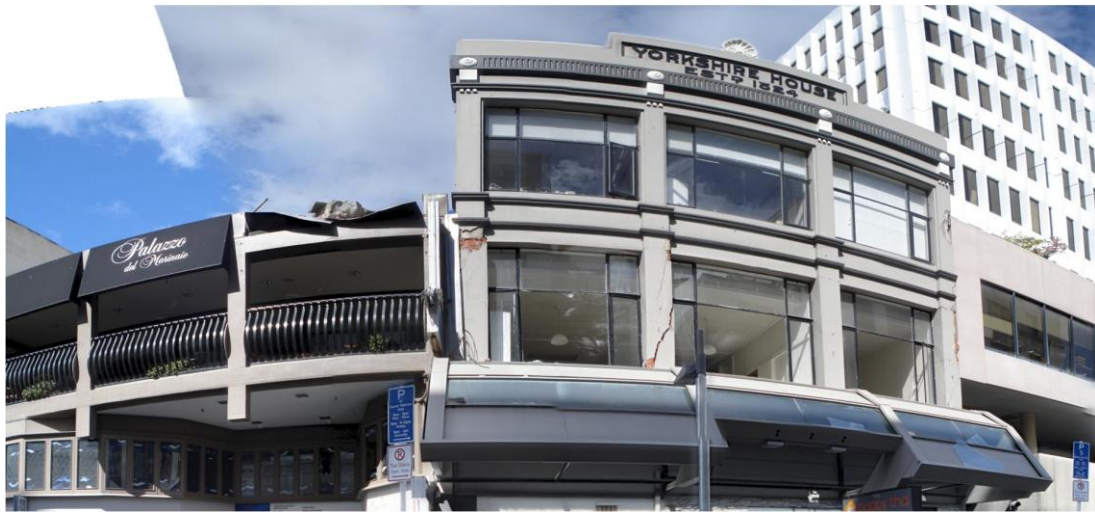
Figure 5: Pounding damage caused by buildings with greatly differing heights. Note image is distorted due to panoramic photography.
