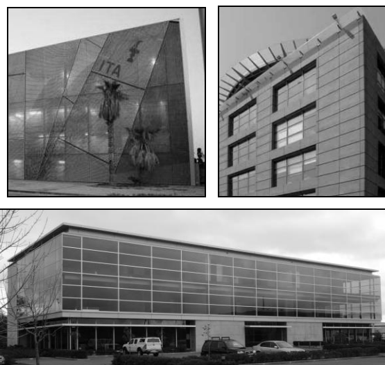
Figure 3: Cladding panel technology; clockwise from top left: double skin, cladding panels, stick curtain.
