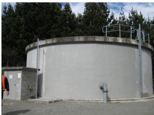
*Figure 1: Reinforced concrete tank.*
