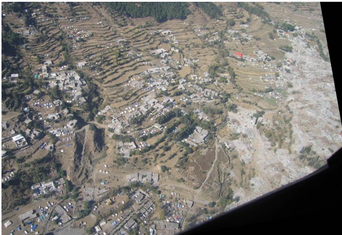
Figure 5. In the town of Balakot building damage is strongly asymmetric and probably delineates the zone of fault rupture. In the area on the right (on the hanging wall) almost every building collapsed, while in the area on the left (on the footwall) ~1 in 10 buildings collapsed.
