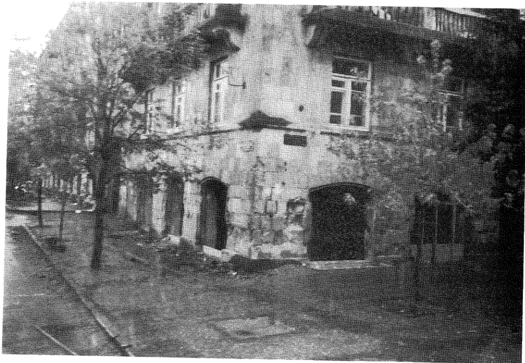
Figure 24 Building in which spread footings were being extended.
