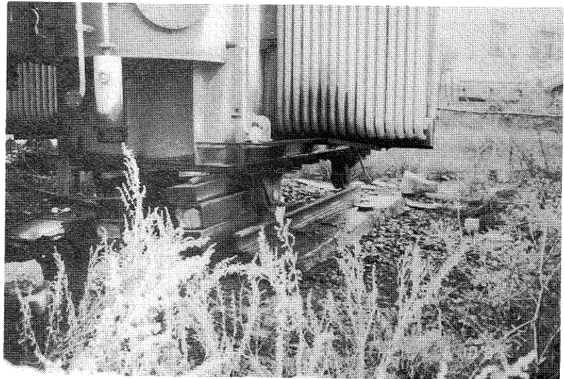
Figure 41 Transformer at Spítak jumped off track.
