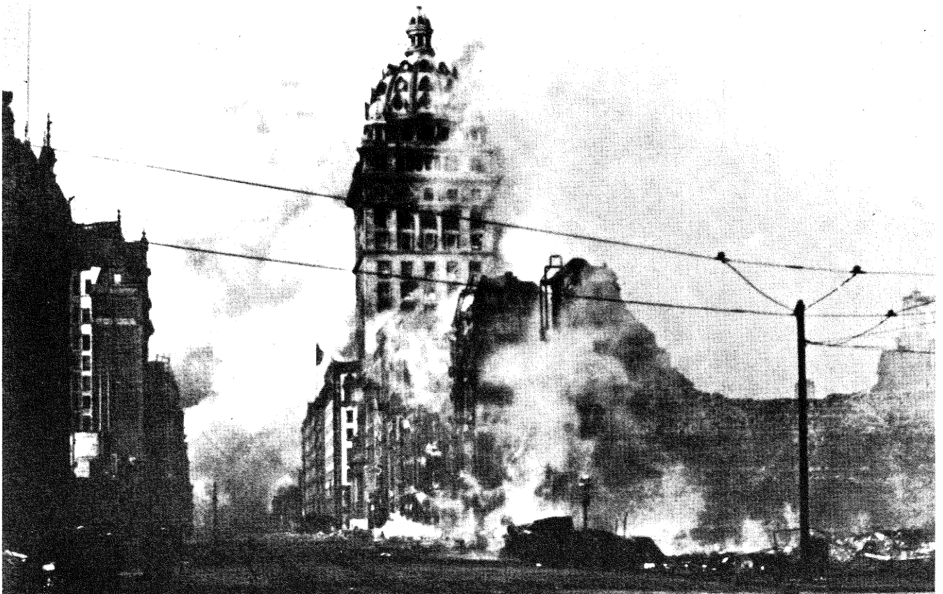
Fig. 3—Market Place, San Francisco and the Call Building after the earthquake of 1906, and during the subsequent fire.
