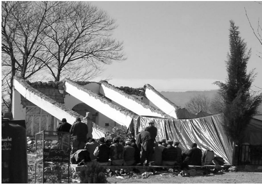
Figure 31. Strong beams weak joint and columns.
