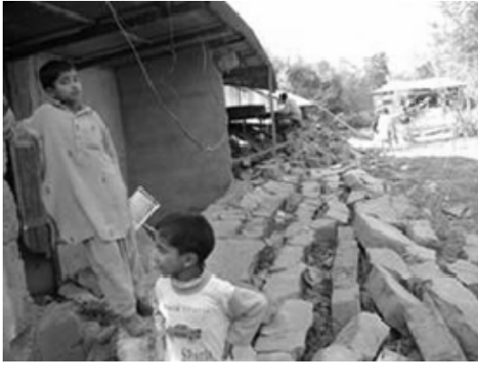
a). Out-of-plane failure of a block wall.
