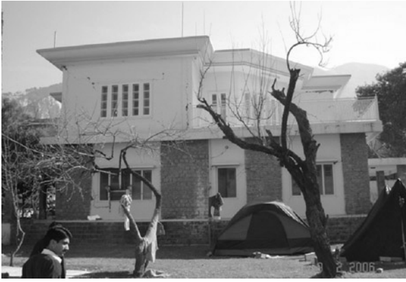
a). A block masonry building in Muzzaffarabad.
