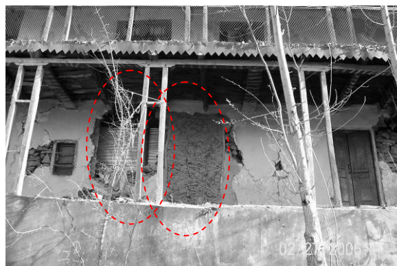
b). Dhaji-dewari portion of wall is intact.
