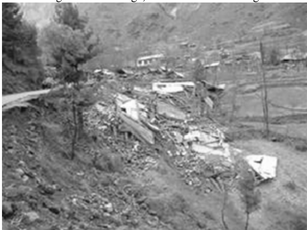
a). Total destruction of buildings constructed on the slope.
