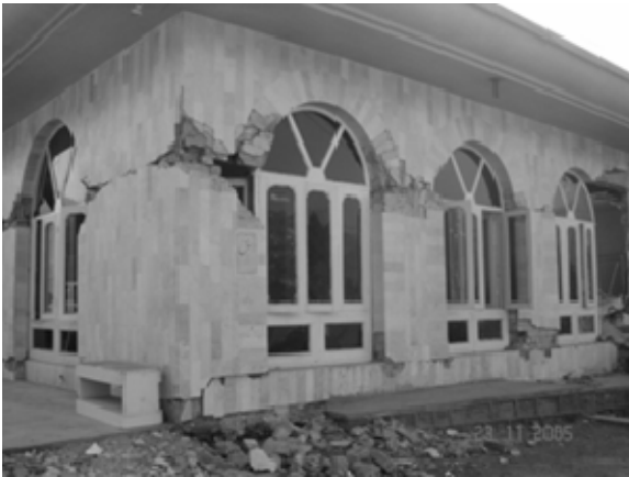
a). Out-of-plane failure of a block wall.
