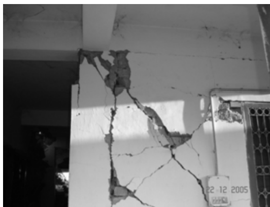
c). Failure of column due to shear forced by infill wall.
