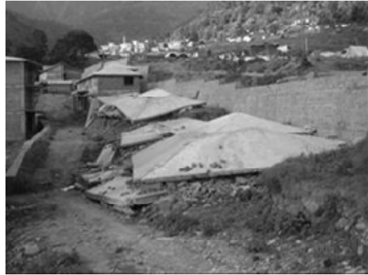
b). Excellent behaviour of hipped RC roof.
