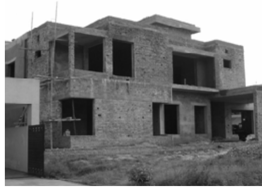
Figure 9. A typical brick masonry building (in the lightly-hit area).
