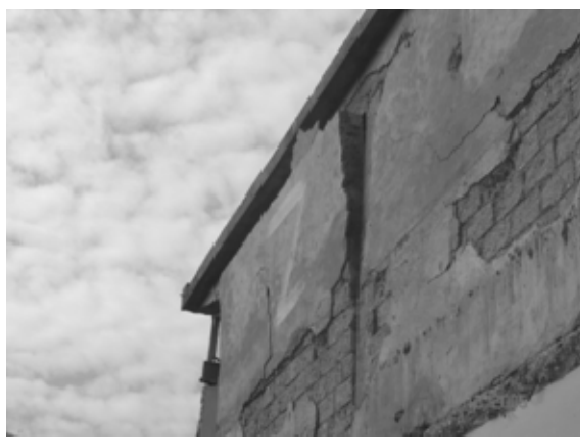
c). Failure of column due to shear forced by infill wall.
