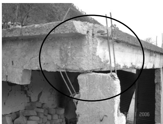
a). Failure of column bar splicing.
