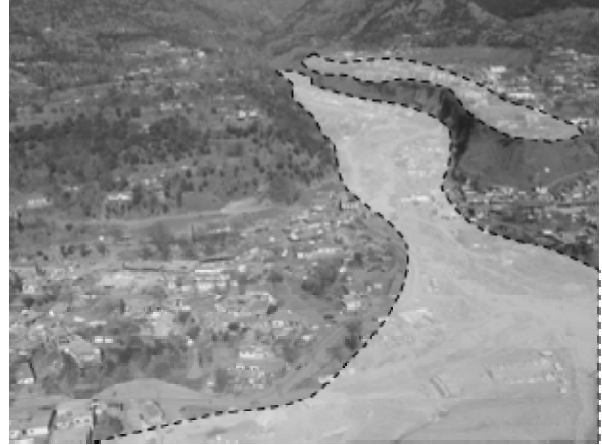
b). Flooding, rockfall and landslide hazard, Bagh, PAK.
