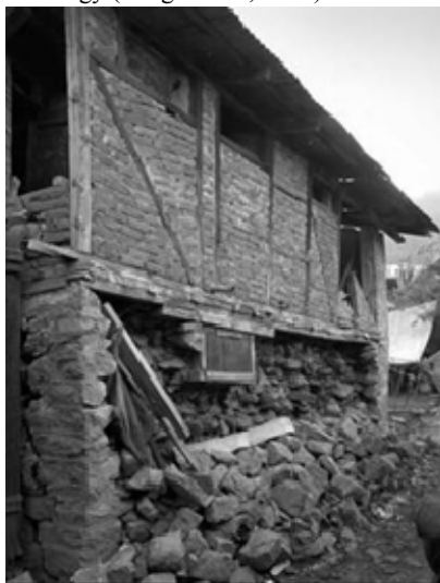
a). Integrity of Dhajji-dewari (Langenbach, 2008).
