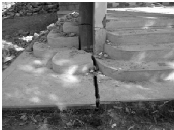
Figure 18. Expression of soil spreading in the form of cracks in floor and walls of houses.
