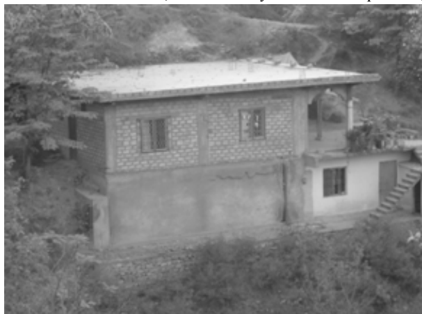
a). A building abutting hill slope survived without much damage.
