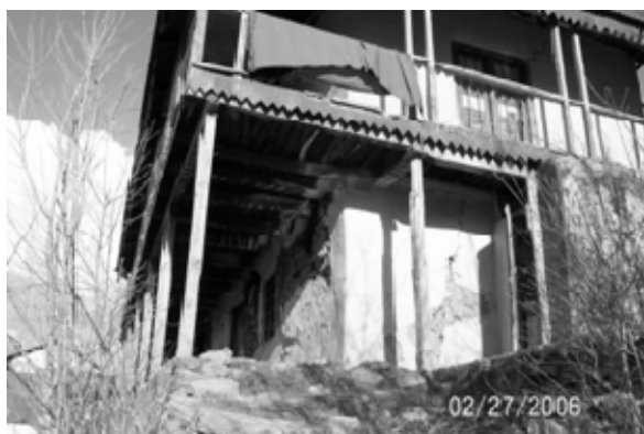
Figure 23. On top of ridge near Rangla, Bagh. No damage at all – presumably due to good configuration.
