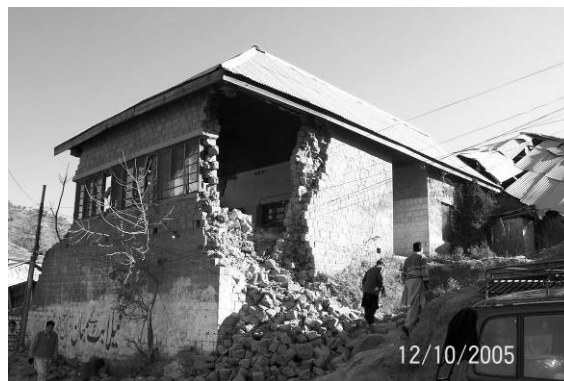
b). Stone masonry with timber truss roof and corrugated iron sheets.
