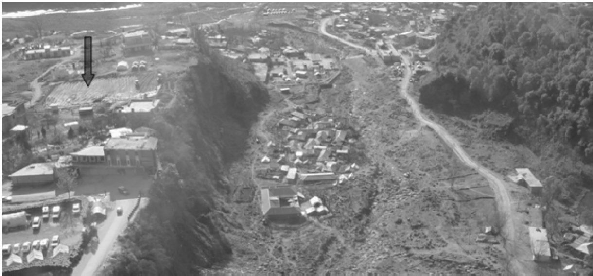
c). Cliff edge, falling hazards, flood plane in Bagh, AJK (site being prepared for a hospital, early 2006).
