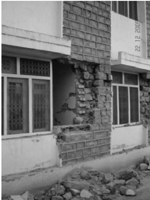
c). Mixing of materials, stone, brick and concrete.
