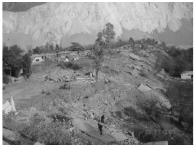
Figure 3. Total destruction of a military camp north of Muzaffarabad. Note the roof slabs thrown off the buildings and an earthquake induced landslide in background across Neelum River. The landslide dammed the river.
