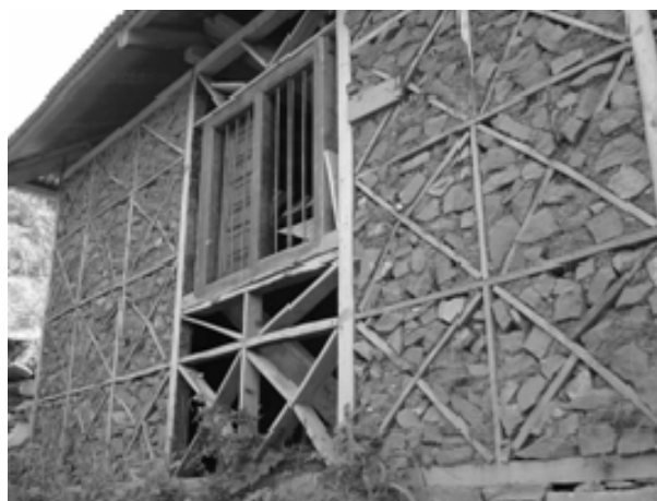
b). Dhajji-dewari under construction.
