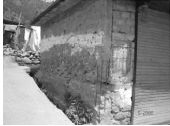
b). A building in plum concrete.
