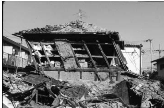
Figure 33. Global instability of timber building.
