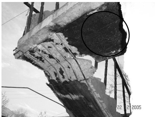
c). Ripping off of the waist slab reinforcement..
