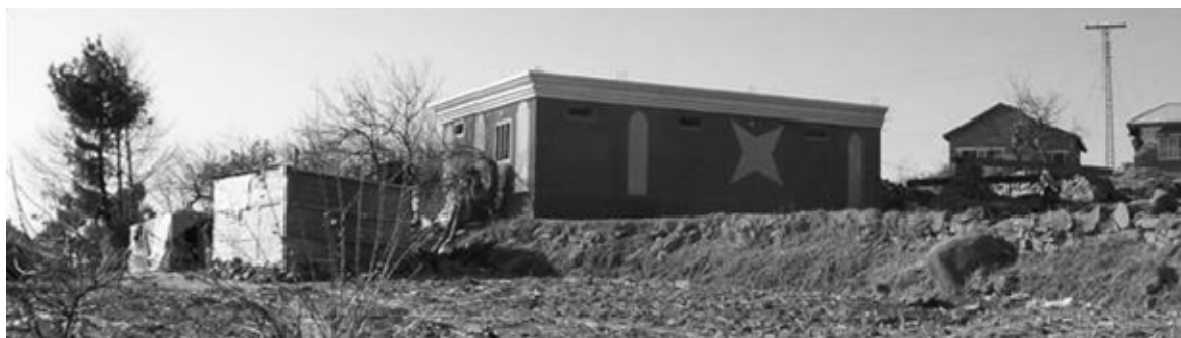
Figure 23. On top of ridge near Rangla, Bagh. No damage at all – presumably due to good configuration.
