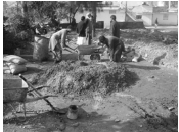
b). Hand-mixing of concrete.
