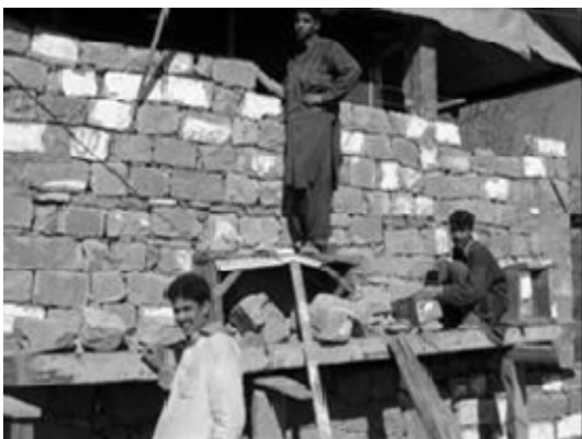
b). Semi-dressed dry stone wall construction after earthquake (also, very tall).
