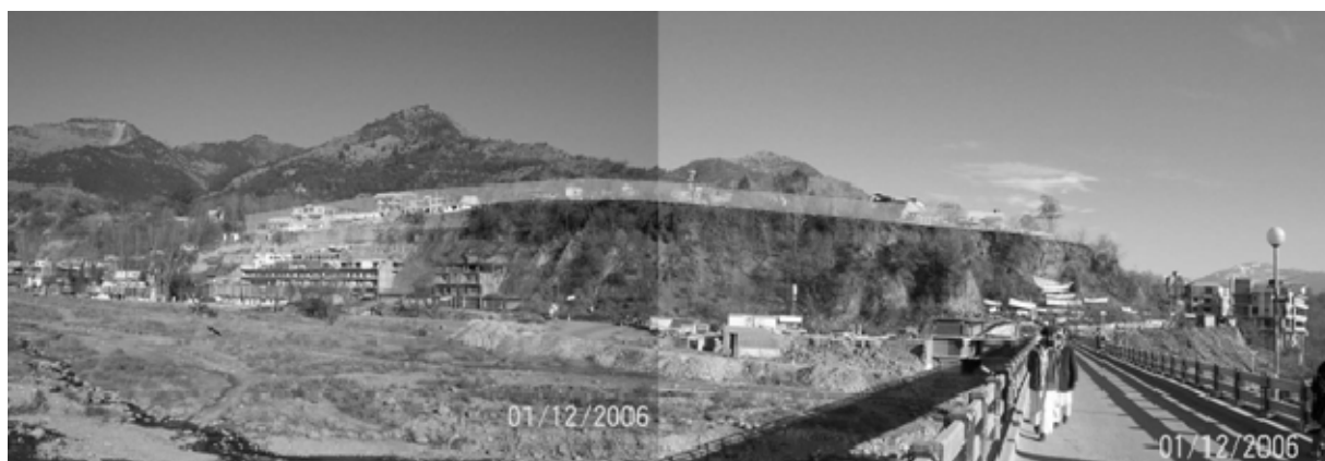
Figure 20. Entire Bagh town edge is built next to unsupported, unstable ground.
