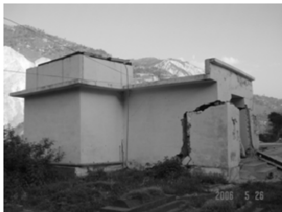
Figure 18. Expression of soil spreading in the form of cracks in floor and walls of houses.
