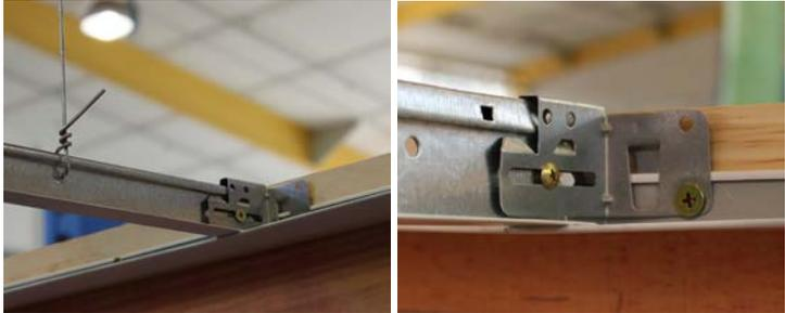
**Figure 3. ACM7 clip installed on tee.**
