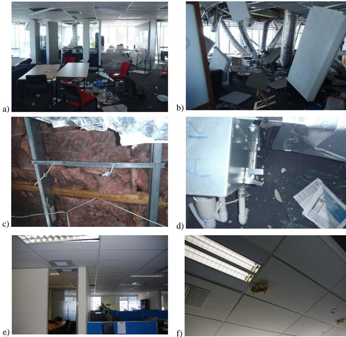
**Figure 2. Observed damage to overhead NSEs following the Canterbury Earthquakes; a) dislodged ceiling tiles and glass partition, b) HVAC unit fallen through ceiling, c) HVAC supports failed, d) failure of HVAC unit fixing, e) distortion of ceiling grid from wall, f) damage to ceiling tiles around sprinkler heads.**
