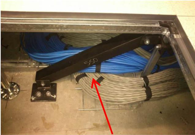
**Figure 8. Sub-floor bracing added to proprietary false flooring.**
