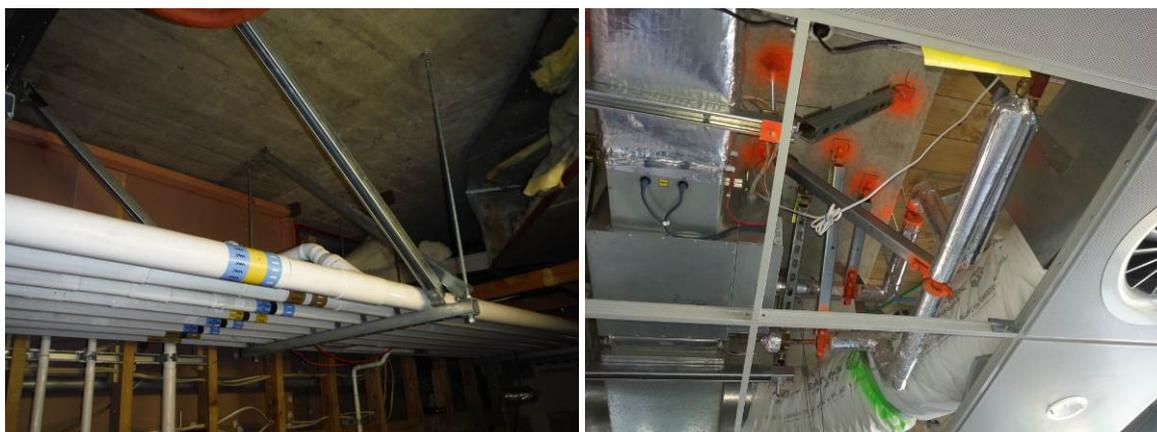
**Figure 1. Restraint of new pipework in an existing building on a single trapeze to reduce the number of braces required (left) and restraint of existing pipework in a modern building (right).**
