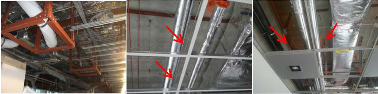
**Figure 9. Vertical inverted portals designed to brace ceiling (left), seismic clips retrofitted to ceiling grid (centre), and ceiling hangers relocated to provide adequate clearance to services (right).**
