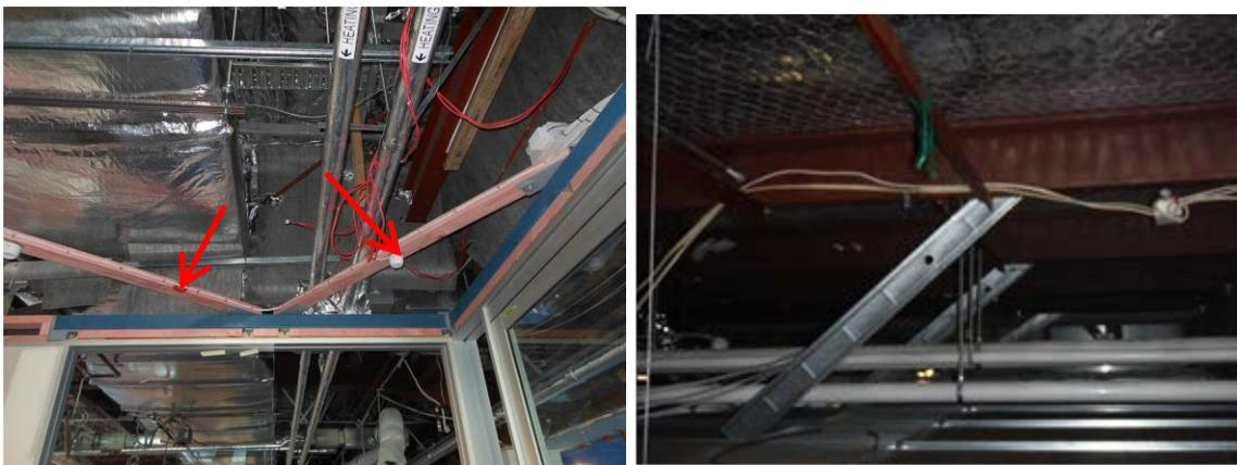
**Figure 10. Horizontal bracing above ceiling level (left), restraint of timber partition wall at ceiling level to primary steelwork using tension/compression brace (right)**
