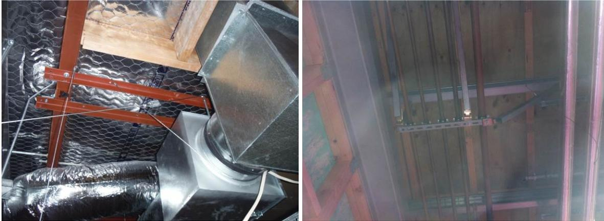
**Figure 4. Cable bracing fixed to secondary steelwork and roof purlins (left) and proprietary rigid bracing in the transverse and longitudinal directions fixed to roof purlins (right).**
