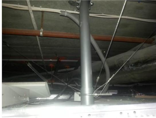
**Figure 2. Wire cables added to brace A.V. equipment above ceiling level.**
