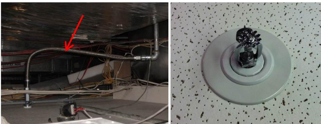
**Figure 6. Compliant flexible sprinkle pipe fixed to ceiling tiles (left), escutcheon cover plate (right)**
