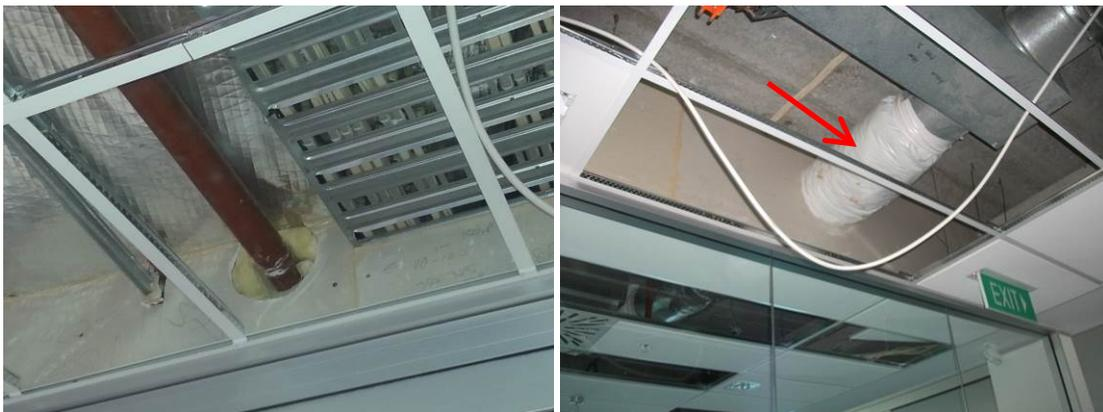
**Figure 5. Rigid services passing through a wall utilising an oversized hole (left), or flexible duct (right).**
