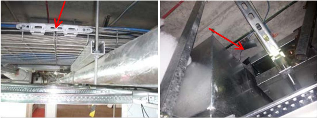
**Figure 7. Proprietary seismic clip added to cable tray to strengthen splice (left), wire tether on HVAC kit (right).**
