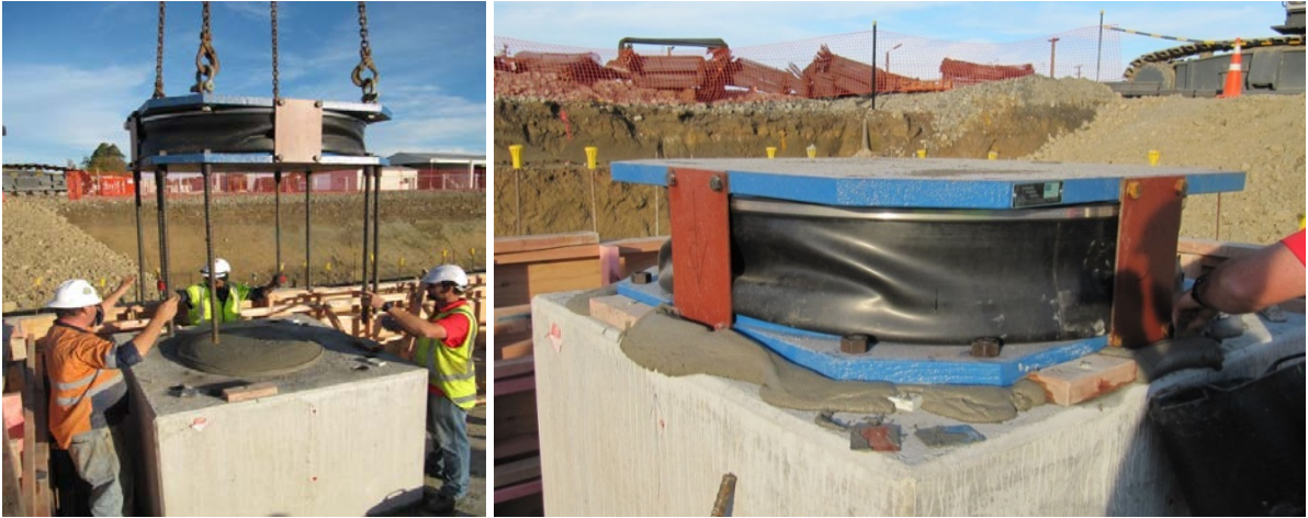
Figure 7. EPS bearing installation
