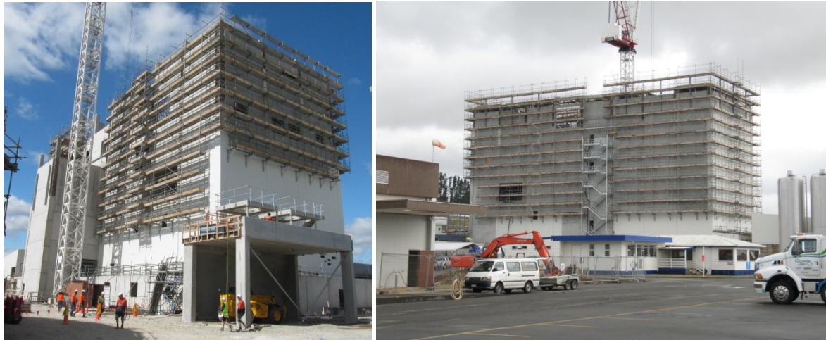
Figure 1. External view of dryer tower building during construction.
