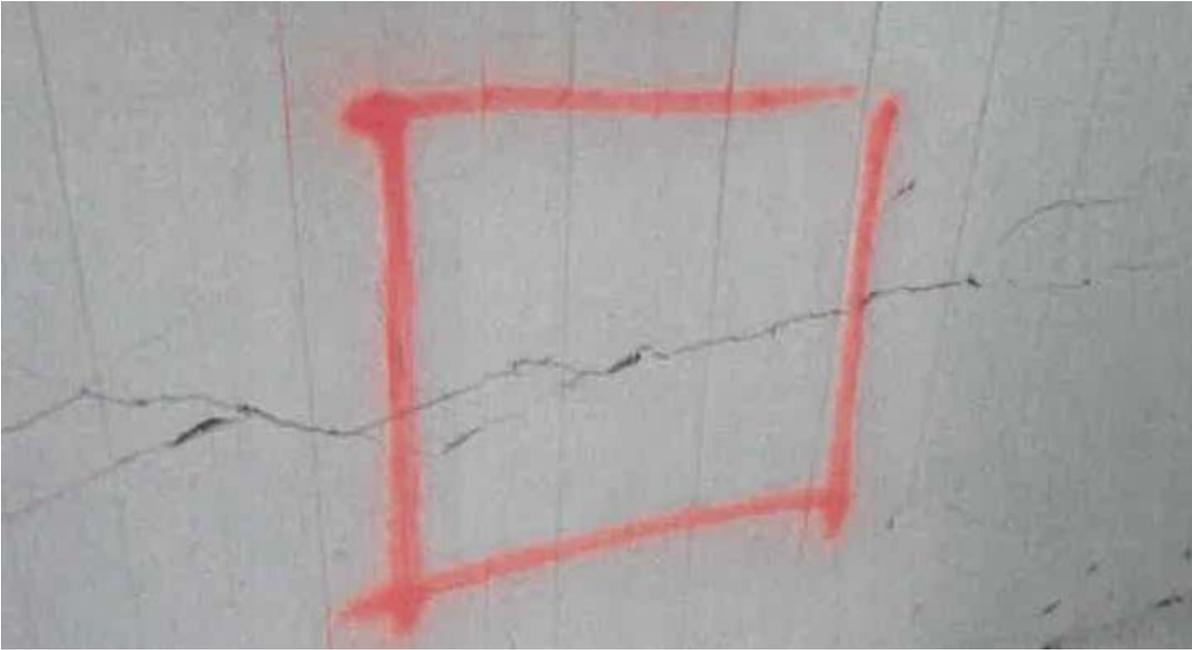
**Figure 1. Cracks in a reinforced concrete structural wall.**
