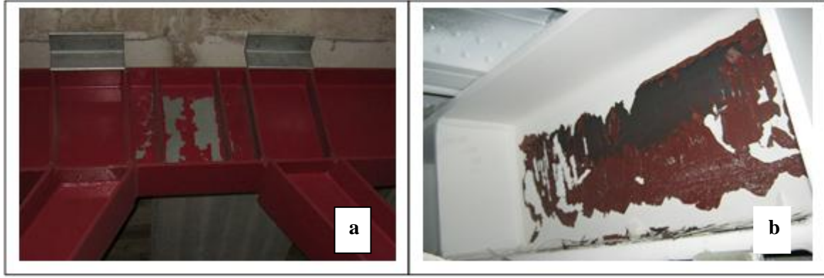
Figure 4.4 Active link beams undergone plastic strain (a) Active link beam at CDHB building, Christchurch (b) Active link beam at Club Tower, Christchurch
