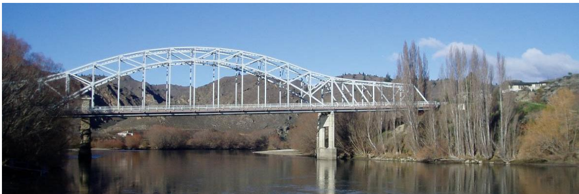
Figure 1: General view of the Clutha River Bridge
