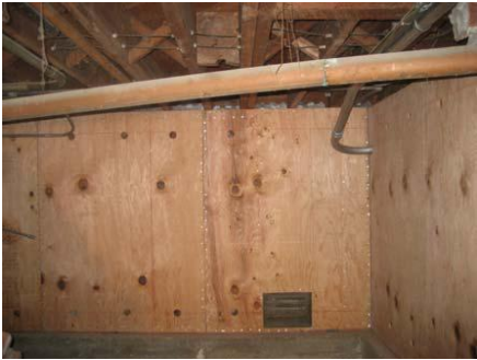
Figure 5: Timber shear wall for retrofit (ATC 2009)
