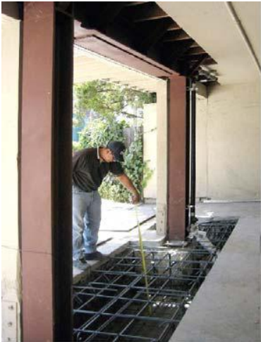
Figure 4: Steel moment-resisting frame for retrofit (ATC 2009)
