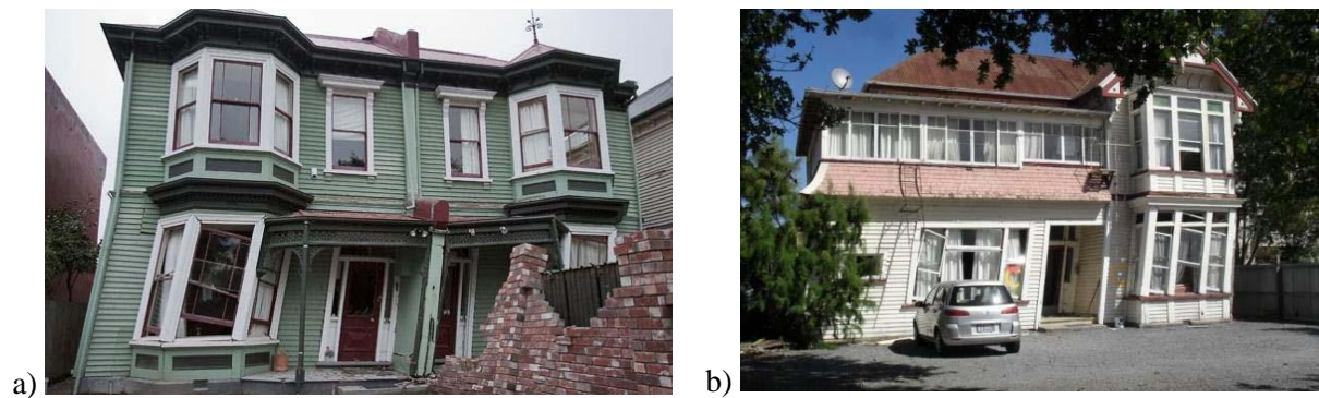
Figure 2: Soft first story observed in Christchurch earthquake (Buchanan 2011)
