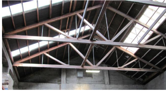
Figure 11: Example of flexible roof diaphragm.
