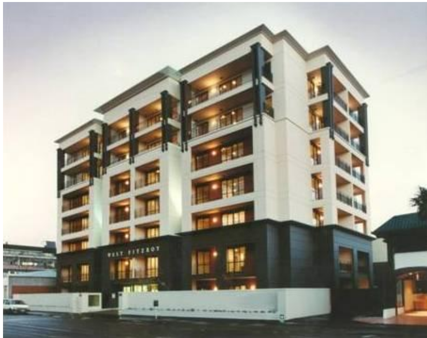
Figure 1. The seven-storey West Fitzroy Apartments building in central Christchurch is an example of a multi-storey tilt-up building which has performed exceptionally well during the Canterbury Earthquakes
