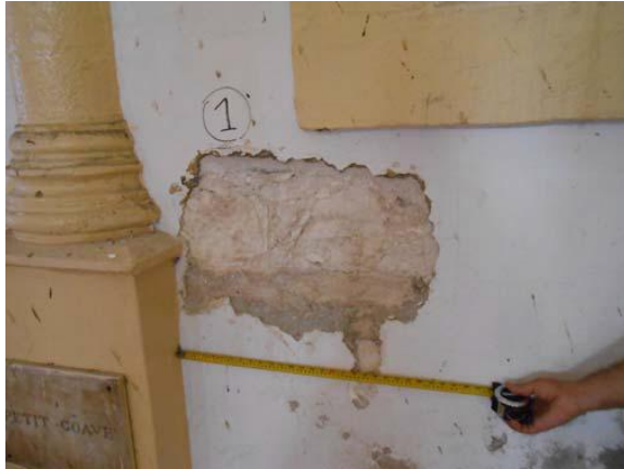
Irregular-shaped stones placed in the mortar
