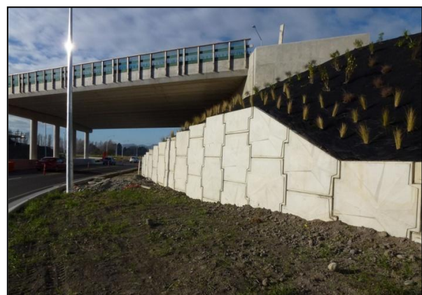
Figure 3: Curletts Road Overpass. West Abutment looking towards the south.
