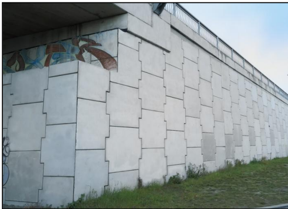
Figure 1: Blenheim Road Bridge. Junction between Walls 1 and 2 (NE corner of bridge).
