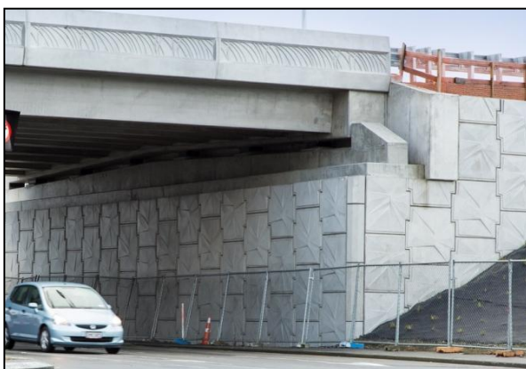
Figure 2: Barrington Street Overpass. SE Corner.
