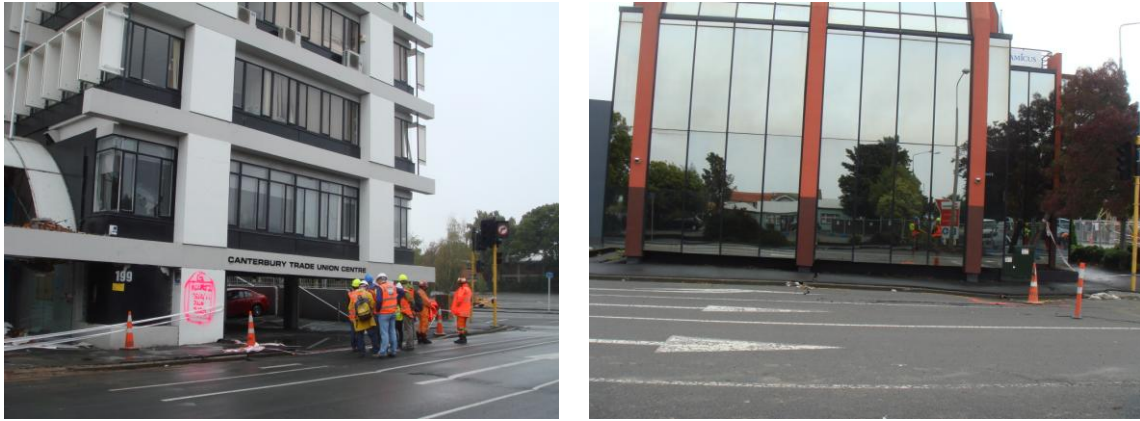
Figure 1: Differential settlement and tilting of structures during the 2011 Christchurch earthquake.
