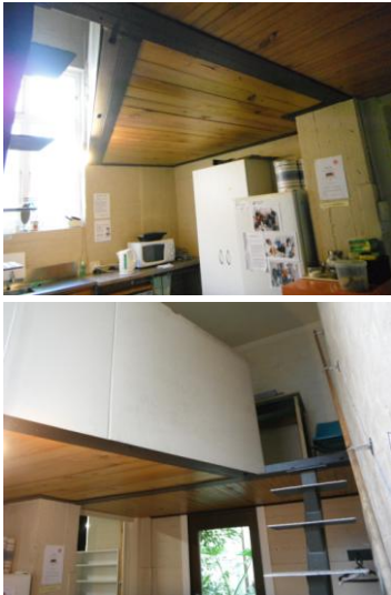
Figure 11. An elevated floor space in a building is irregularly shaped and connected to the surrounding structure eccentrically.
