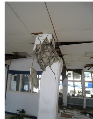
Figure 3. Plastic hinge formed in non-ductile column-sway mechanism.
