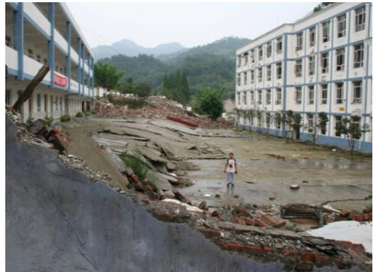
Figure 2. School destroyed by landslide (left); Collapsed school building across ruptured fault (right)
