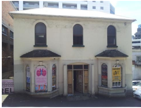
(a) View of Southern wall (2012)
