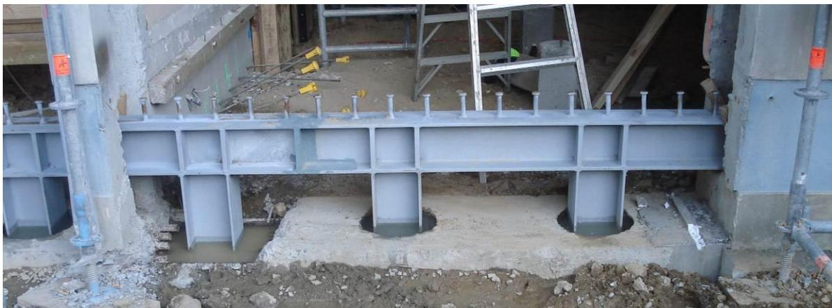
To allow for the additional displacements imposed by this flexible and ductile system, all longitudinal beams that framed into rotating elements were “pinned” as below.
