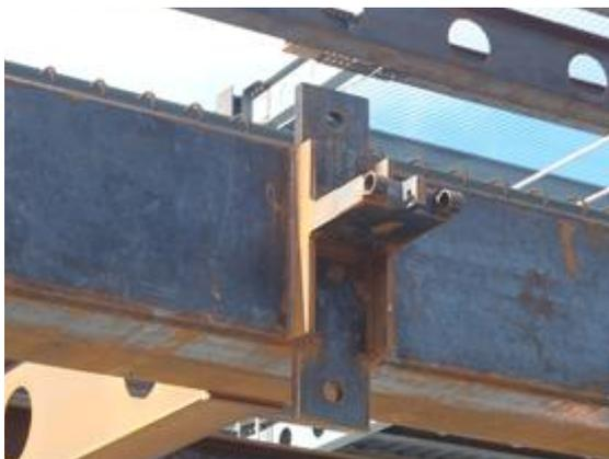
**Figure 8:** Tongue plate protruding from floor structure that slots through the seismic frame
