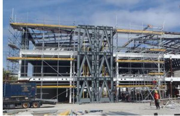
**Figure 7:** Pair of steel braced frames erected on-site.
