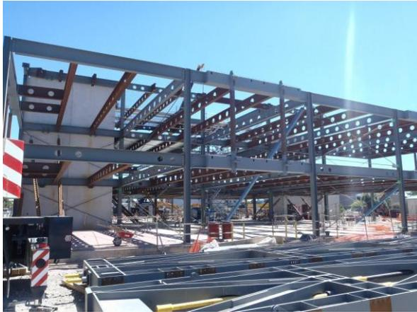
**Figure 10:** Concrete-steel composite floor structure under construction
