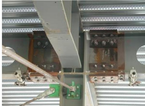
**Figure 11:** Sliding Hinge Joint utilised for secondary frames
