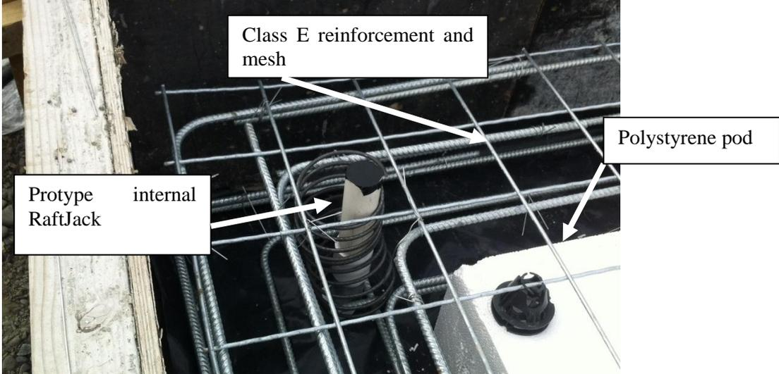
Figure 3 internal jacks prior to pouring concrete
