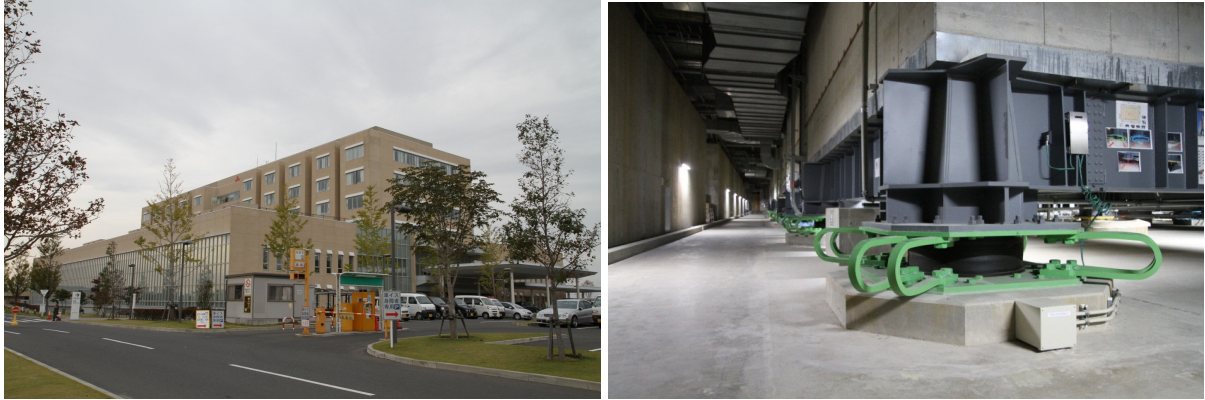
Figure 1. Ishinomaki Red Cross Hospital [left] and detail of the seismic isolation devices (rubber bearings coupled with U-shaped steel dampers) [right]
